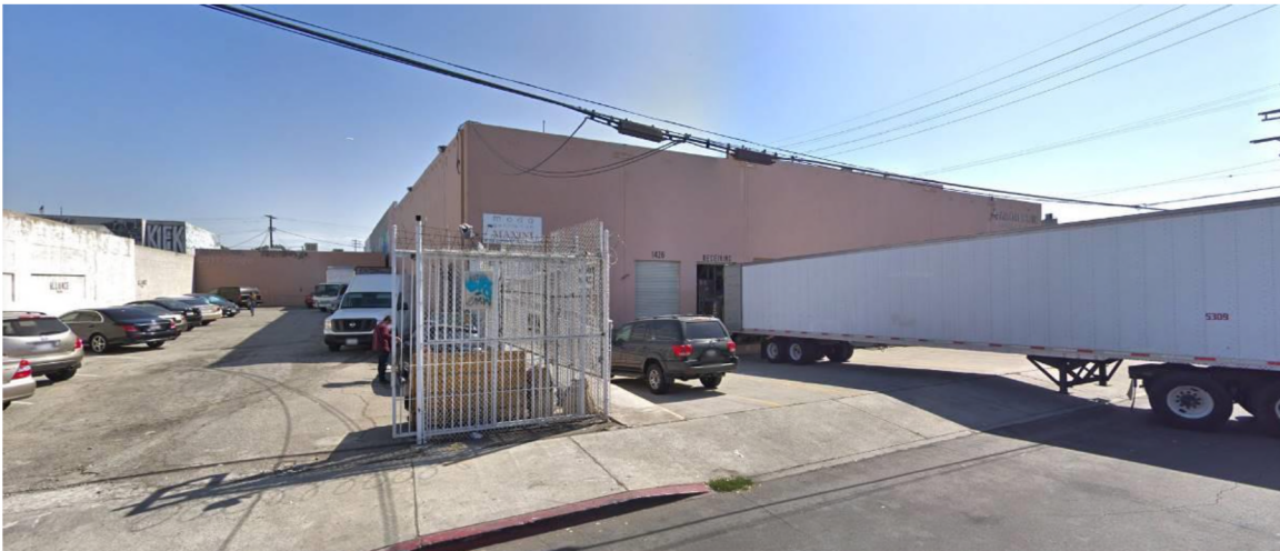
1426 Paloma Street from west. The property includes the open space on the north that also provides access to the building. There is a ramp up from the sidewalk to an entry door.
