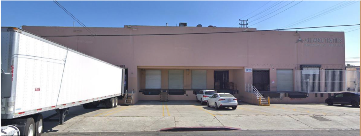
View of Paloma Street elevation. The projects is located in the northerly (left) half of the building. Several of the loading dock openings will be modified and filled in for the project.
