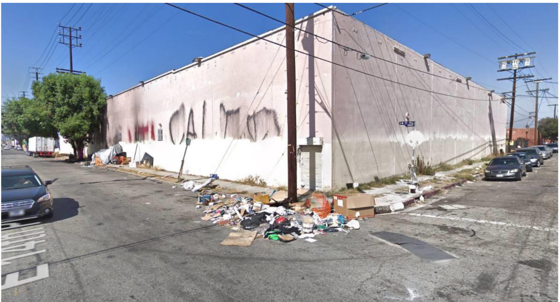
1426 Paloma Street from southeast corner at Essex Street. The walls are blank and windowless.
