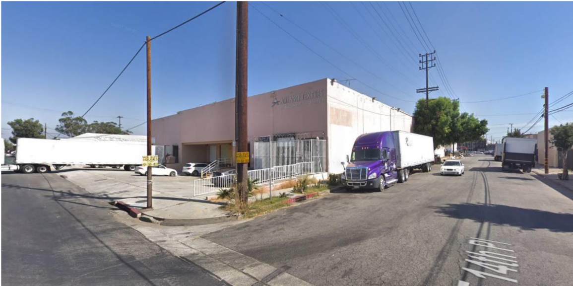
1426 Paloma Street from southwest corner at 14th Place. The building is setback from Paloma Street for loading dock access. A pedestrian ramp leads up to the office area.
