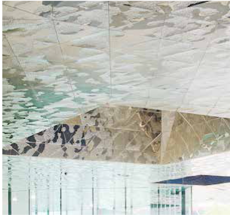
5: STAMPED TEXTURED METAL SOFFIT
