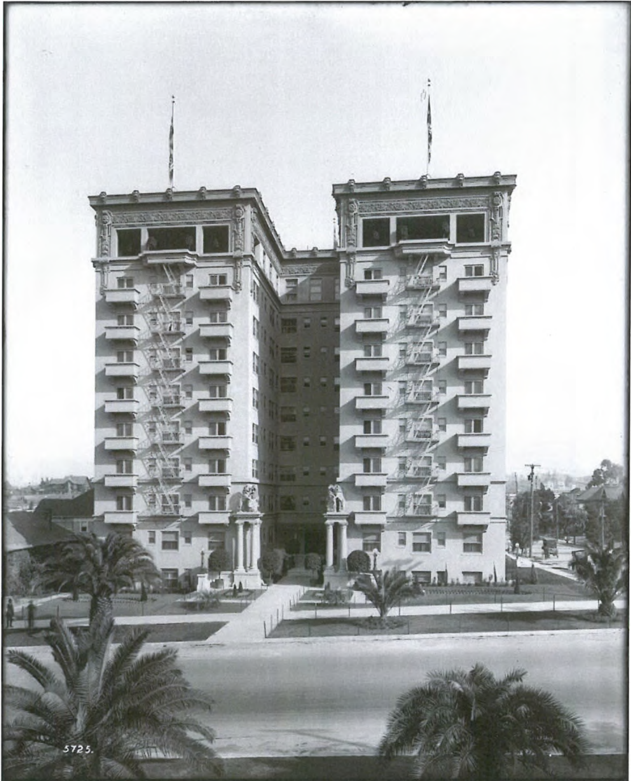
ca. 1917 photograph of the primary (southwest) elevation of the Bryson Apartments. View looking northeast from Wilshire Blvd. (source: USC Digital Library)
