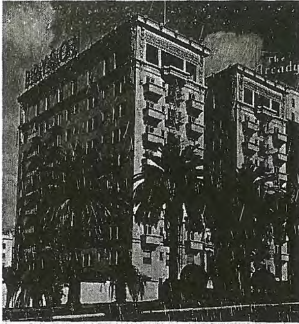
WILSHIRE DOWAGER. —Photo of Bryson Apartment Hotel, 2701 Wilshire Blvd., taken in mid-1940s, shows establishment almost as it looks today, except that palms in front are now much taller.
