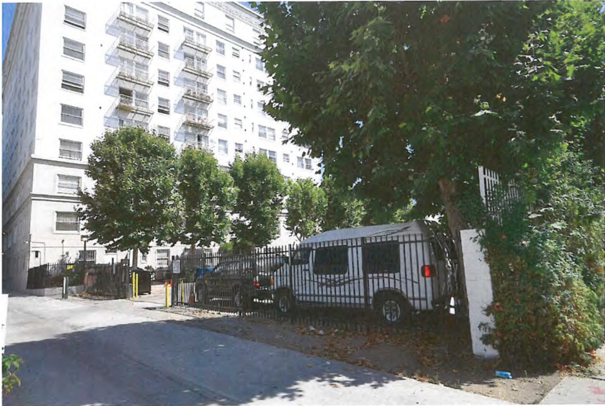
Bryson Apartments, view of southwest elevation and parking lot facing east. (GPA Consulting, July 2019)
