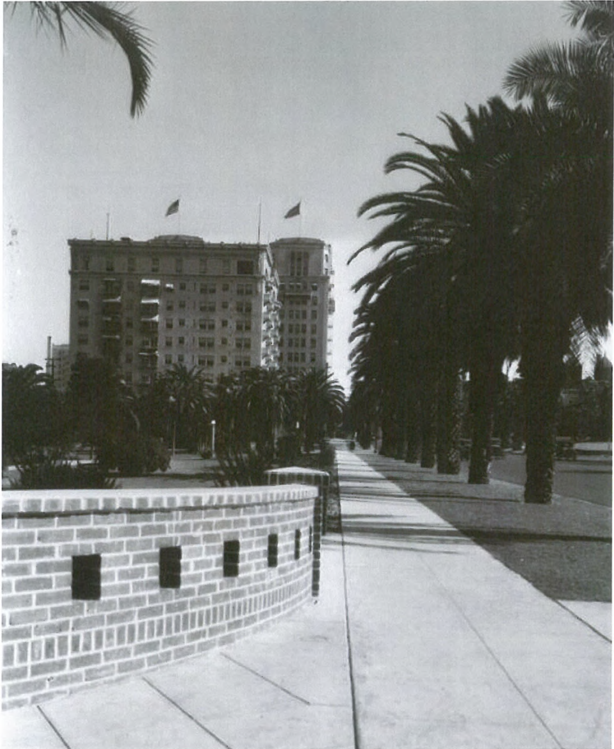
n.d., photograph of the northwest elevation of the Bryson Apartments from Lafayette Park. (source: LAPL)
