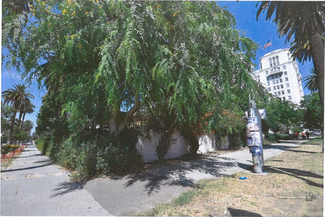
Bryson Apartments, view parking lot facing north. (GPA Consulting, July 2019)
