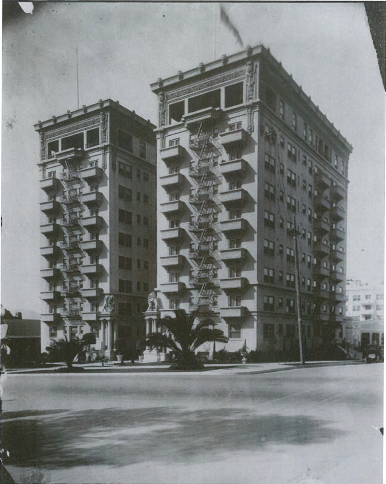
ca. 1913-1915 photograph depicting the Bryson Apartments soon after original construction. View looking north from the intersection of Wilshire Blvd. and S. Rampart Blvd. (source: USC Digital Library)
