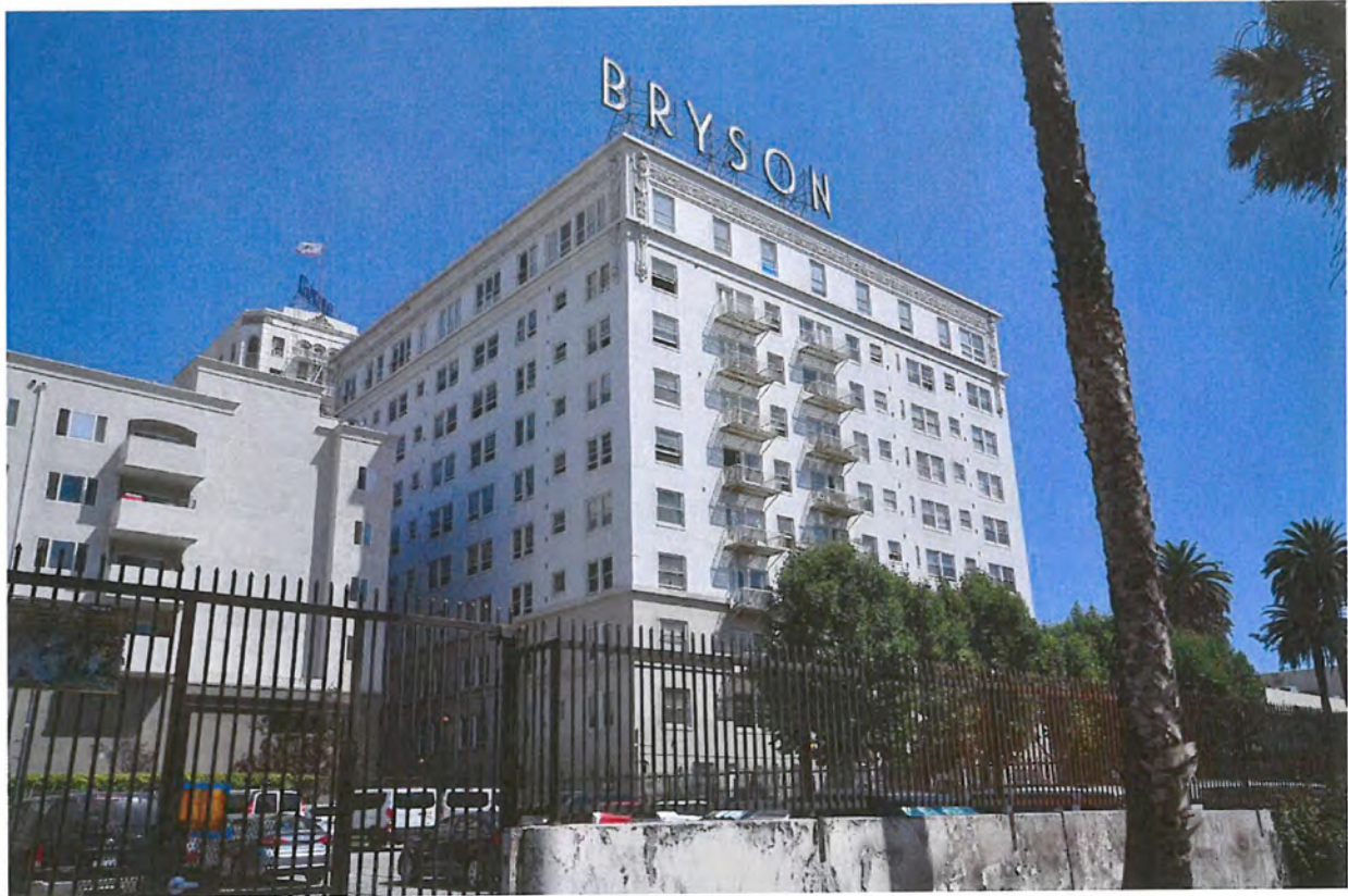
Bryson Apartments, view of northwest and southwest elevations. (GPA Consulting, July 2019)
