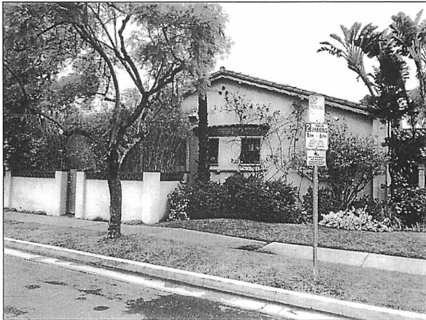
Figure 10. East façade, view west (SWCA, 2019).
