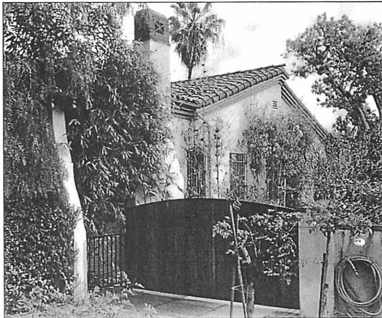
Figure 7. West façade, view southeast (SWCA, 2019).
