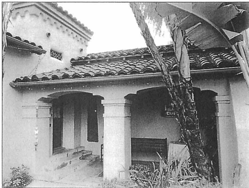
Figure 5. Detail of primary entrance and arcade, view southwest (SWCA, 2019).
