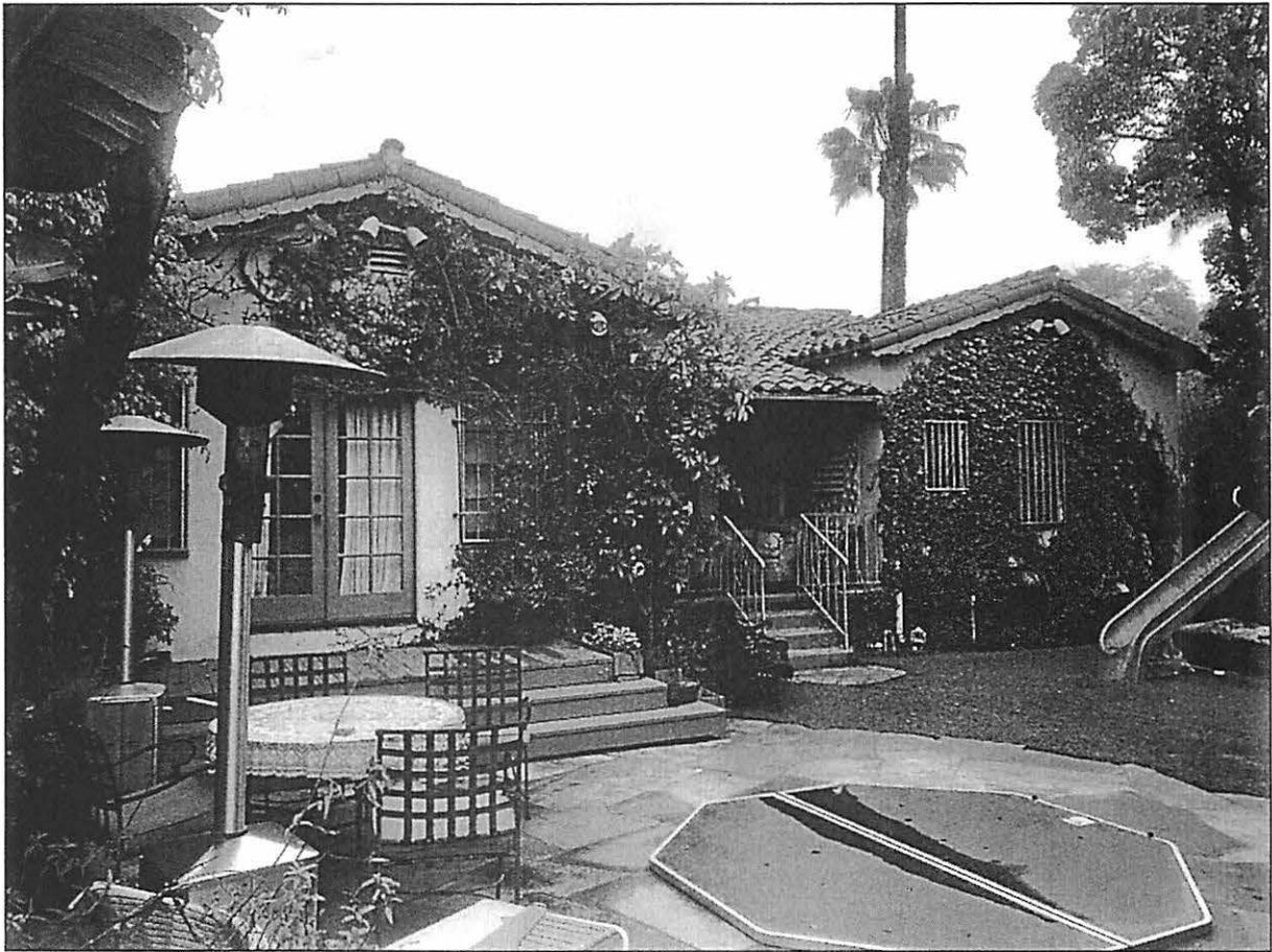
Figure 8. Rear (south) façade, view north (SWCA, 2019).
