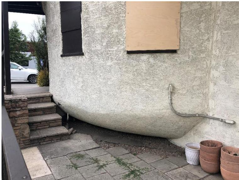
**Figure 8. Detail of Rough Textured Stucco, Brick and Stone Veneer, and Boarded-Up Windows**
