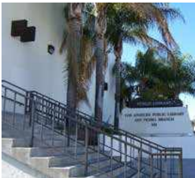
San Pedro Branch Library on Gaffey Street
