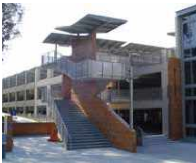
Solar panels on top of parking structure
