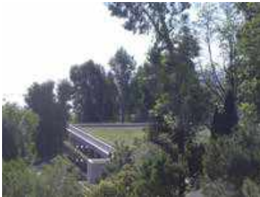
Green roof of a parking structure
