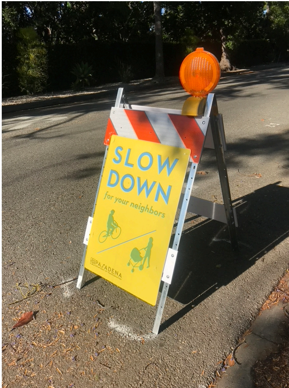
Image 1 - The City of Pasadena has simple, yet high visibility graphic signage for their Safety Streets Measure wherein local streets remain accessible to traffic. Note the markings on asphalt to ensure signs are properly positioned. Some streets have signage located at the curb edge - rather than street center - which functions as a temporary curb extension which has been shown to slow vehicular traffic around corners.
