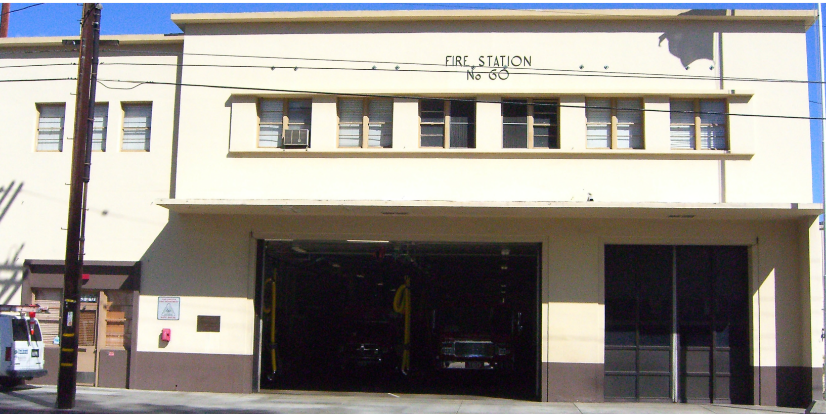
A fire station serving the North Hollywood community.
