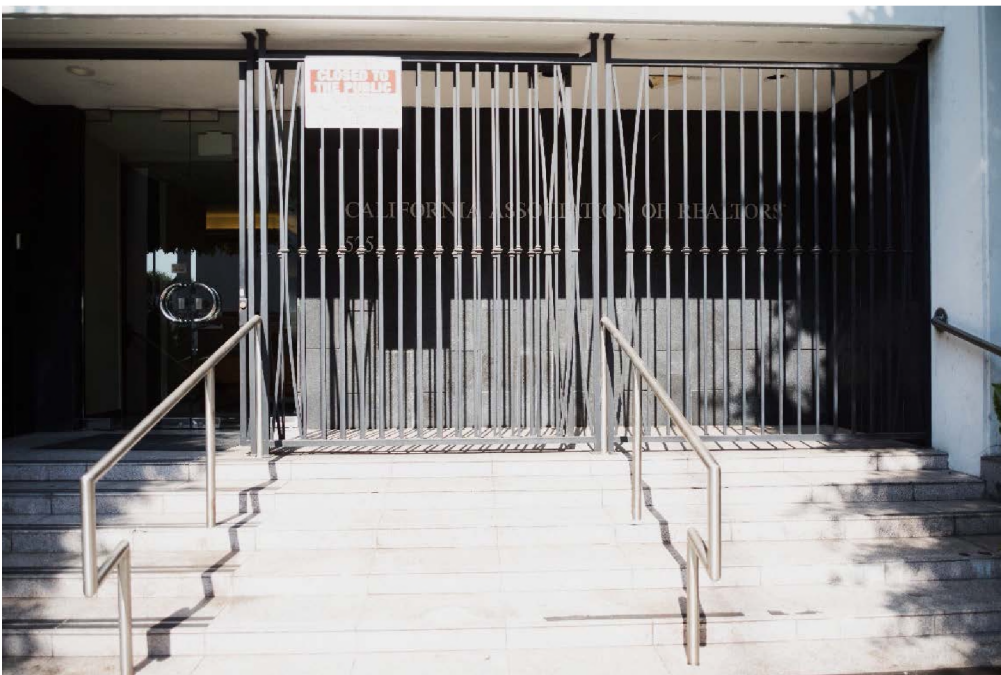
Detail view of primary entrance doors and steps.
