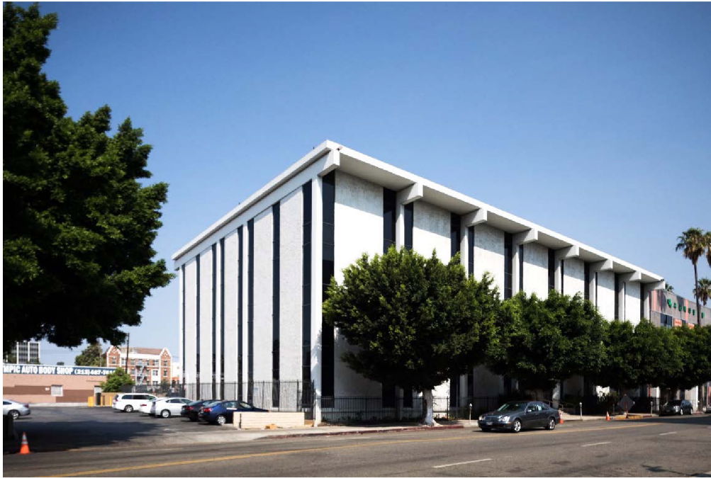
East (primary) and south façades, view facing northwest.
