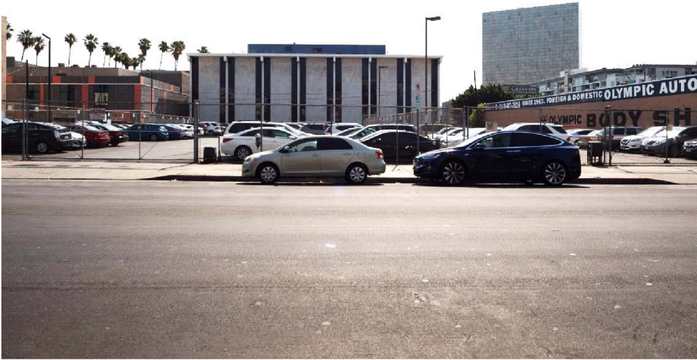
West façade and surface parking lot, view facing east.
