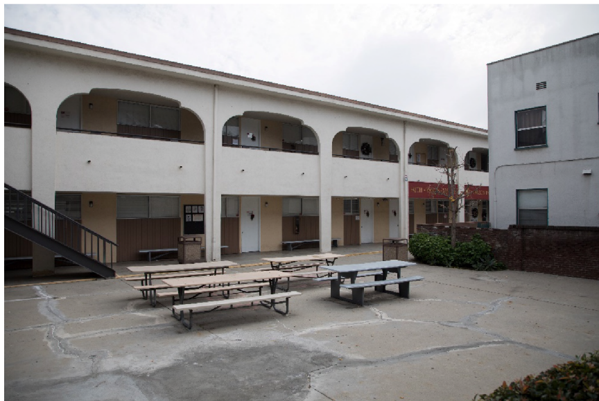
Classroom building, view facing southeast.
