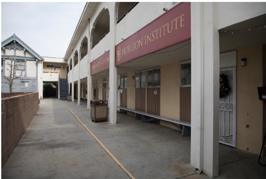
Classroom building and single-family residence, view facing north.
