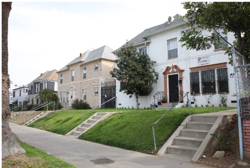
1200 Menlo Avenue (at right), directly north of Project Site, view facing northeast.
