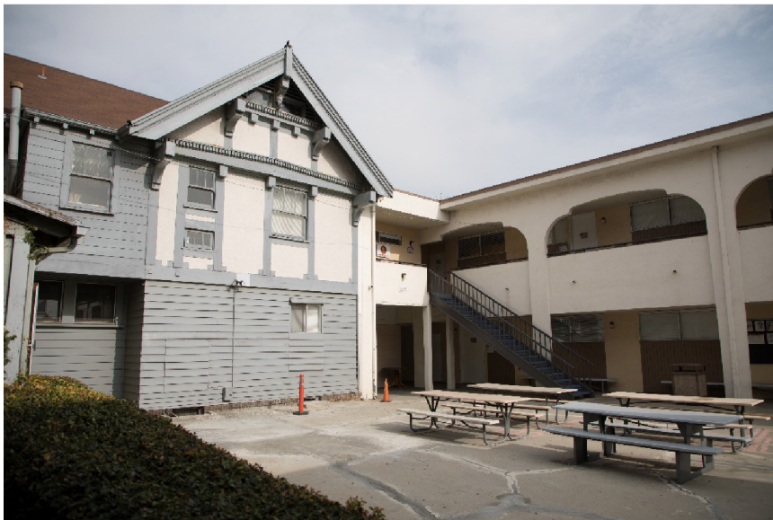
Japanese Language School Unified System/former single-family residence and abutting classroom building, view facing northeast.
