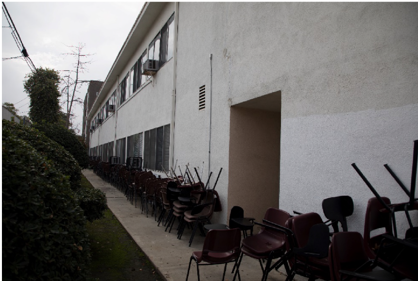
Rear of classroom building, view facing southwest.
