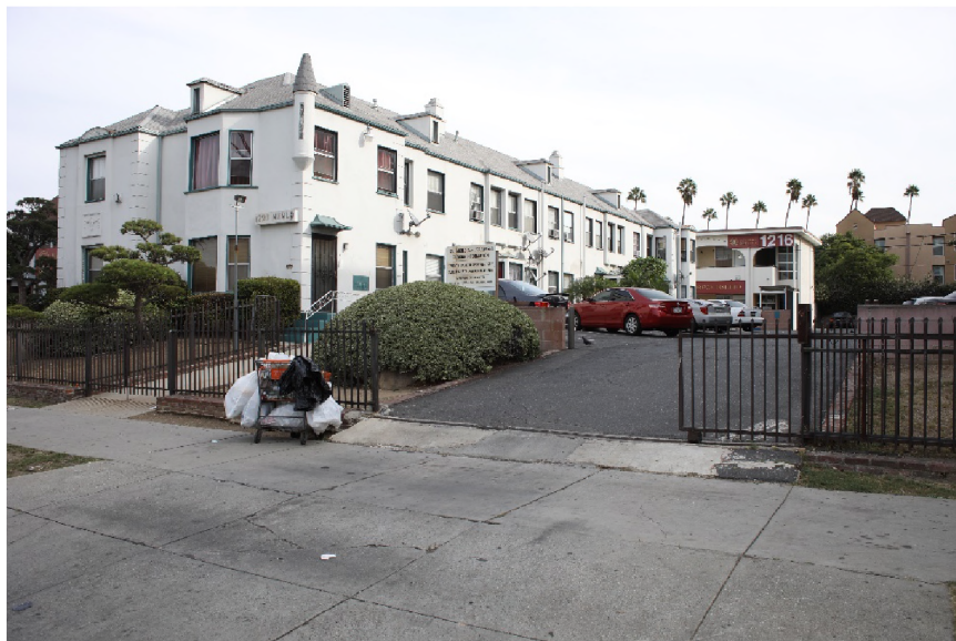
Multi-family residence (1224 Menlo Avenue), view facing northeast.
