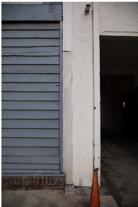
Detail view where the former single-family residence abuts the classroom building.
