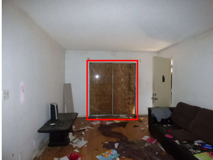
Figure 45 Typical living room in typical apartment unit, view facing east. Addition of plywood sheathing outlined in red
