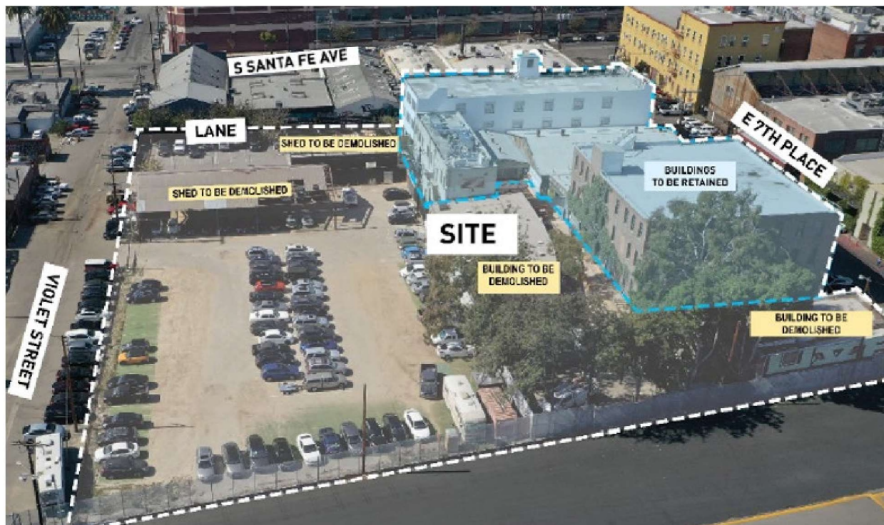
Aerial View of Existing Development
