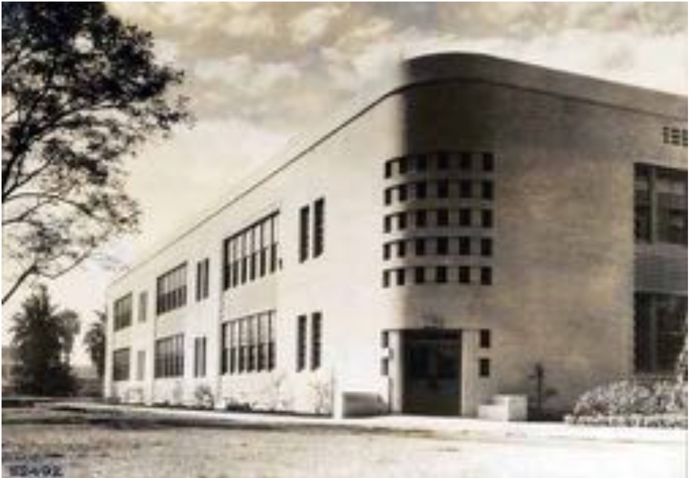
Figure 5: Science Building, 1935. Source: SAIC Digital Libraries, Ryerson & Burnham Archives.
