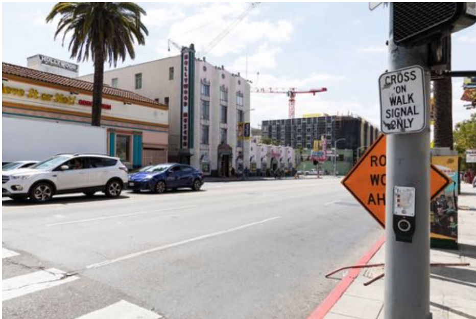
Primary façade of the Max Factor Makeup Salon building, view facing southeast across Highland Avenue.
