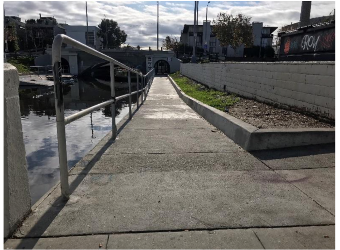
Canal St (W/S), looking Southerly
