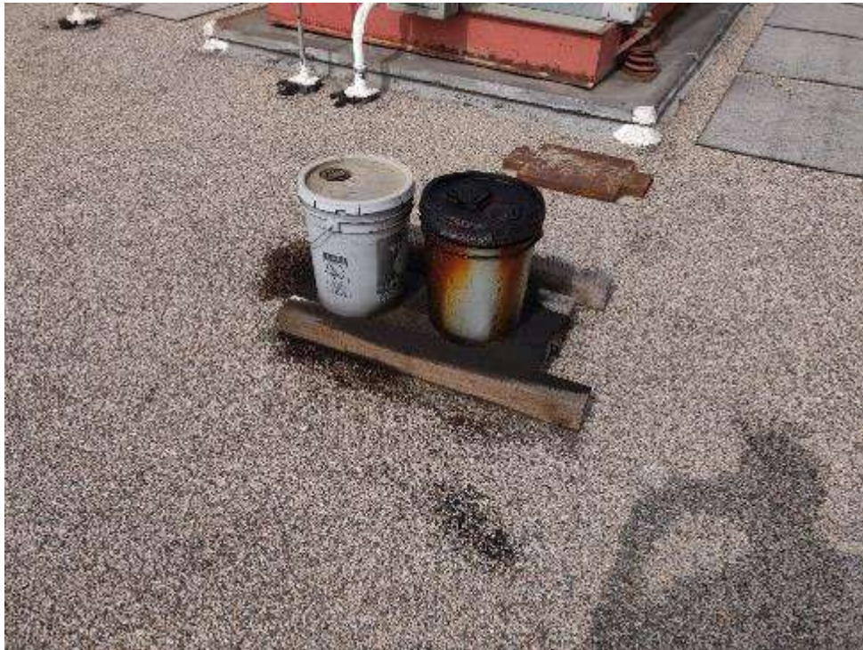
Photo 17: Oil containers with associated de minimis visible staining on the roof of the LA Probation Building (West Block)
