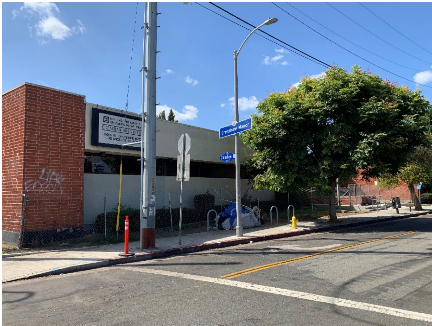
North elevation, facing southwest
