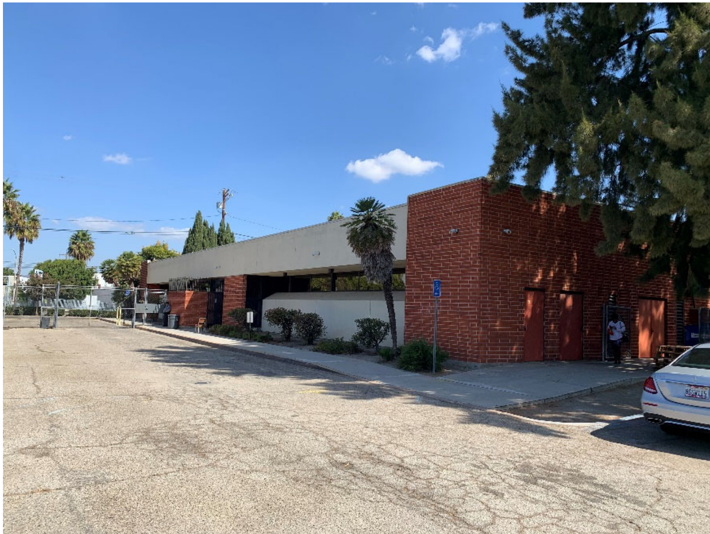
West elevation, facing northeast
