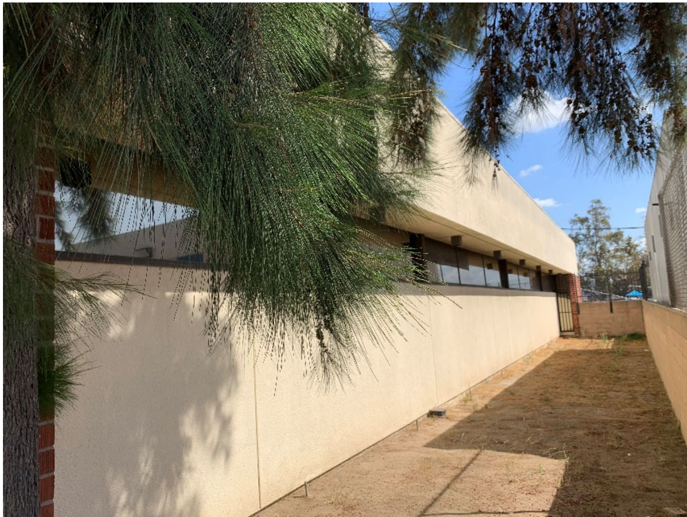
South elevation, facing northeast
