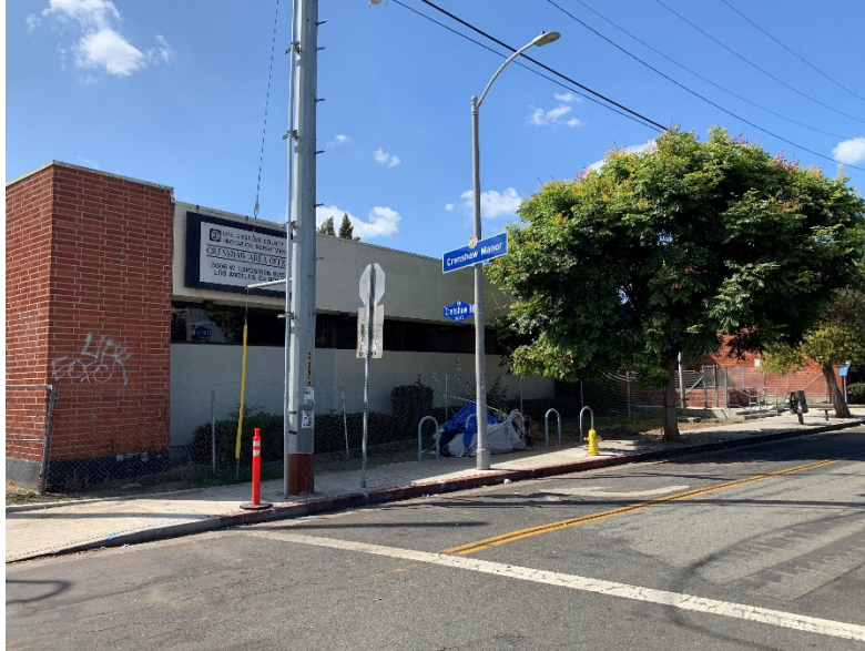
Figure 5-2 North elevation, facing southwest
