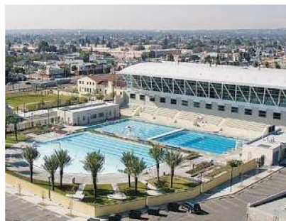
Expo Center Electrification, Efficiency
