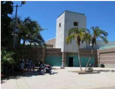
Balboa Sports Complex Electrification, PV, BESS
