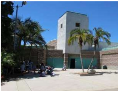
Balboa Sports Complex Electrification, PV, BESS
