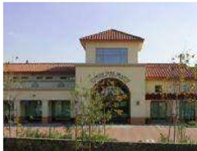
Cypress Branch Library Electrification, Efficiency, PV, BESS
