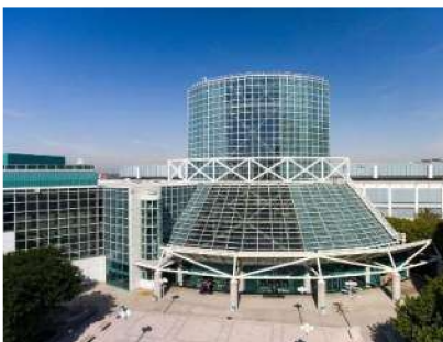
Convention Center Electrification, Efficiency, PV
