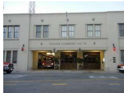
Old Fire Station #39 Electrification, Efficiency, PV, BESS
