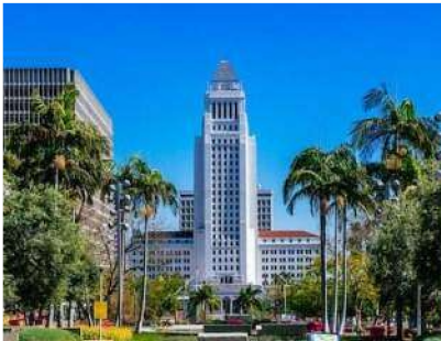
City Hall Electrification, Efficiency
