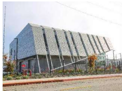
North Hollywood Sewer Yard
