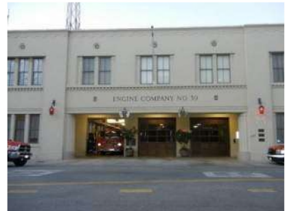
Old Fire Station No. 39 Electrification, Efficiency, PV, BESS
