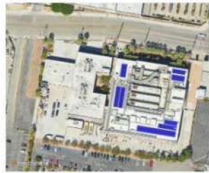
Emergency Operations Center
