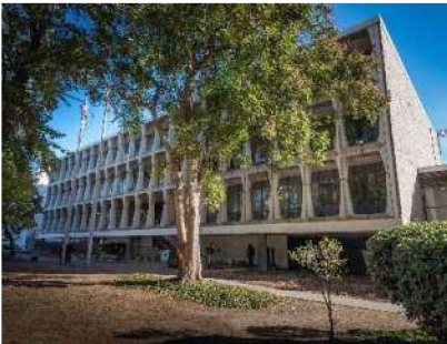
Van Nuys Police Station Electrification, Efficiency
