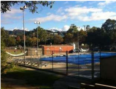
Yosemite Pool + Rec Center Electrification, Efficiency
