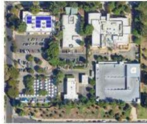
West Valley Municipal Building
