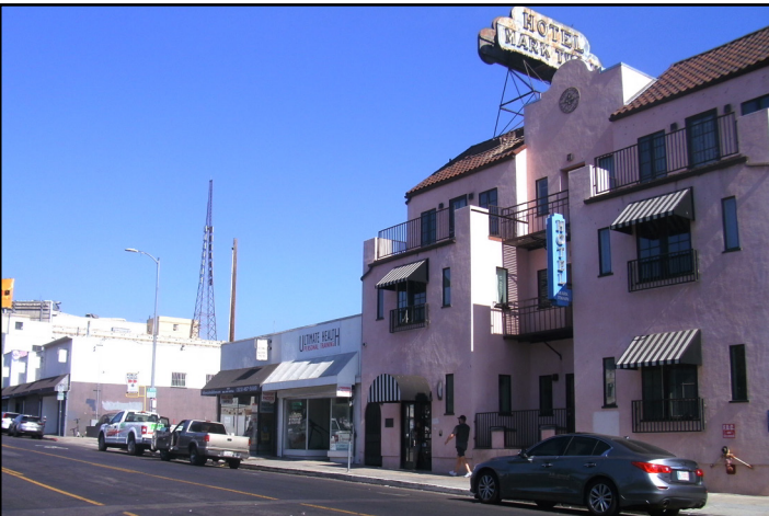
View 11: On the west side of Wilcox Avenue looking northwest at the properties northwest of the Project Site.
