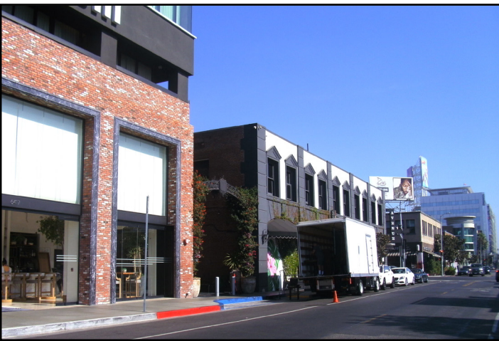
View 9: On the south side of Selma Avenue looking northeast at properties east of the Project Site.
