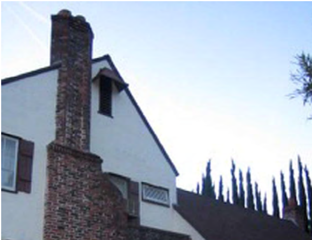
Jablonski Residence, chimney, 1973 Carmen Avenue, 2021 (Multiple listings Photo)
