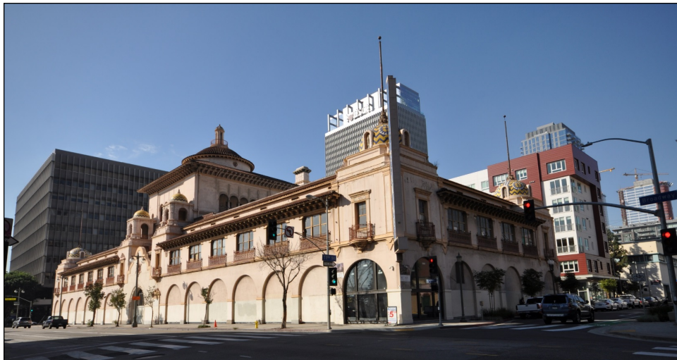
Figure 20: Los Angeles Herald Examiner Building, 1111 S. Broadway (GPA)
