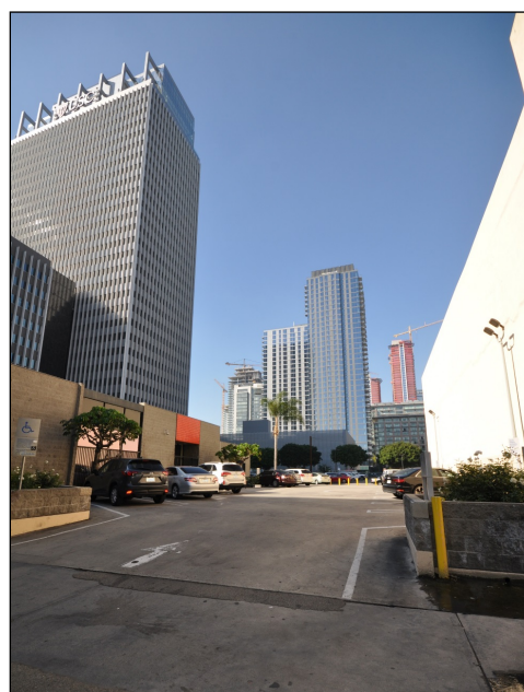
Figure 7: Southern elevation of the Project site building, view facing west toward parking lot and bank building on former site of Southwestern University (GPA)
