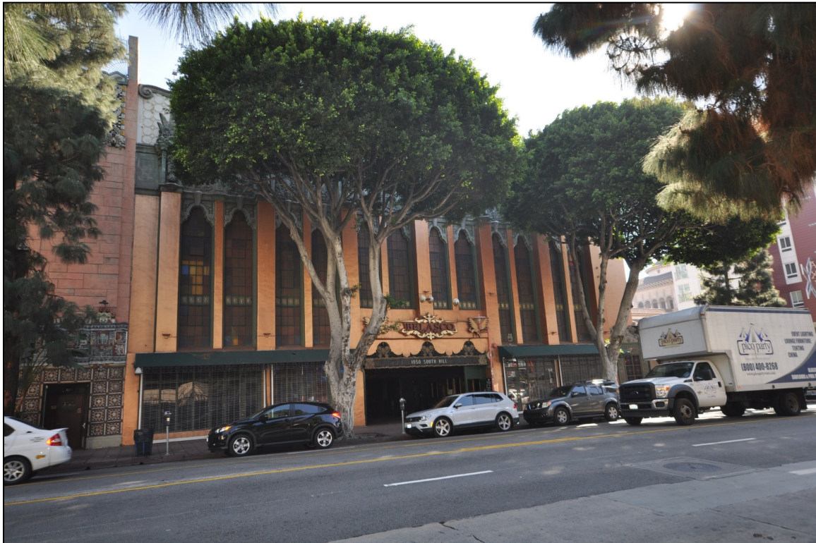
Figure 17: Belasco Theater, 1050 S. Hill Street, view facing east (GPA)
