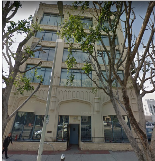
Figure 12: Joseph Basch Company Building, 1031 S. Hill Street, view facing west (Google)
