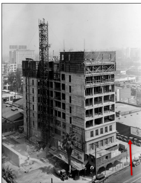
Figure 6: Southwestern University, 1121 S. Hill Street, under construction c. 1930s. The Project site is in the lower right (see arrow). The Project site was developed with the current building in 1954. (Security Pacific National Bank Collection, LAPL)
