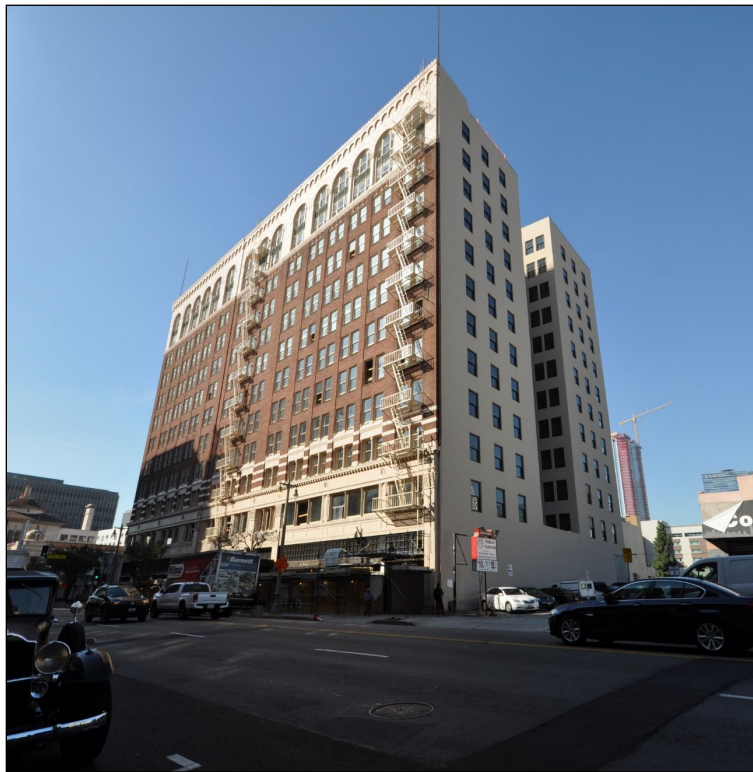
Figure 18: Western Pacific Building, 1023 S. Broadway, view facing southwest, 2018 (GPA)
