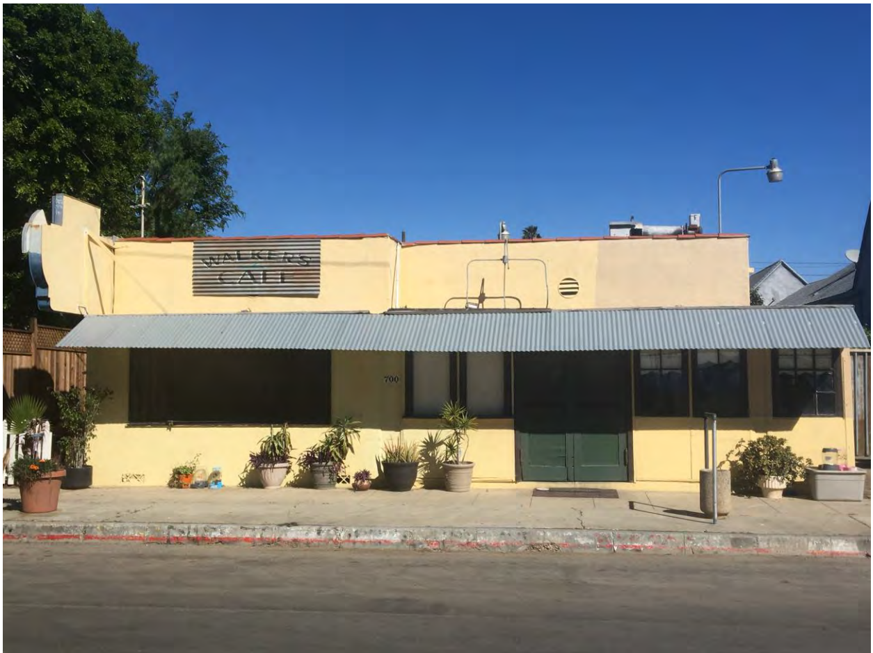
Commission/Staff Site Inspection Photos—February 10, 2022 Page 1 of 5
