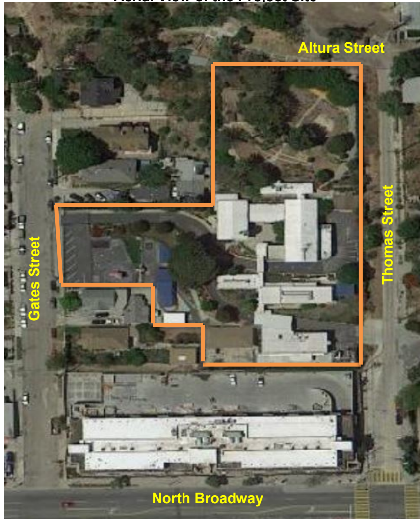
Aerial View of the Project Site
