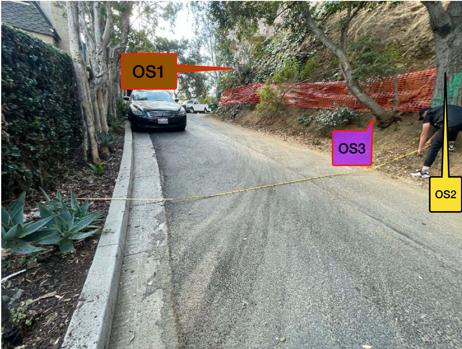
PHOTO 10 - Shows front slope and steep terrain. House will be built directly into hillside.
