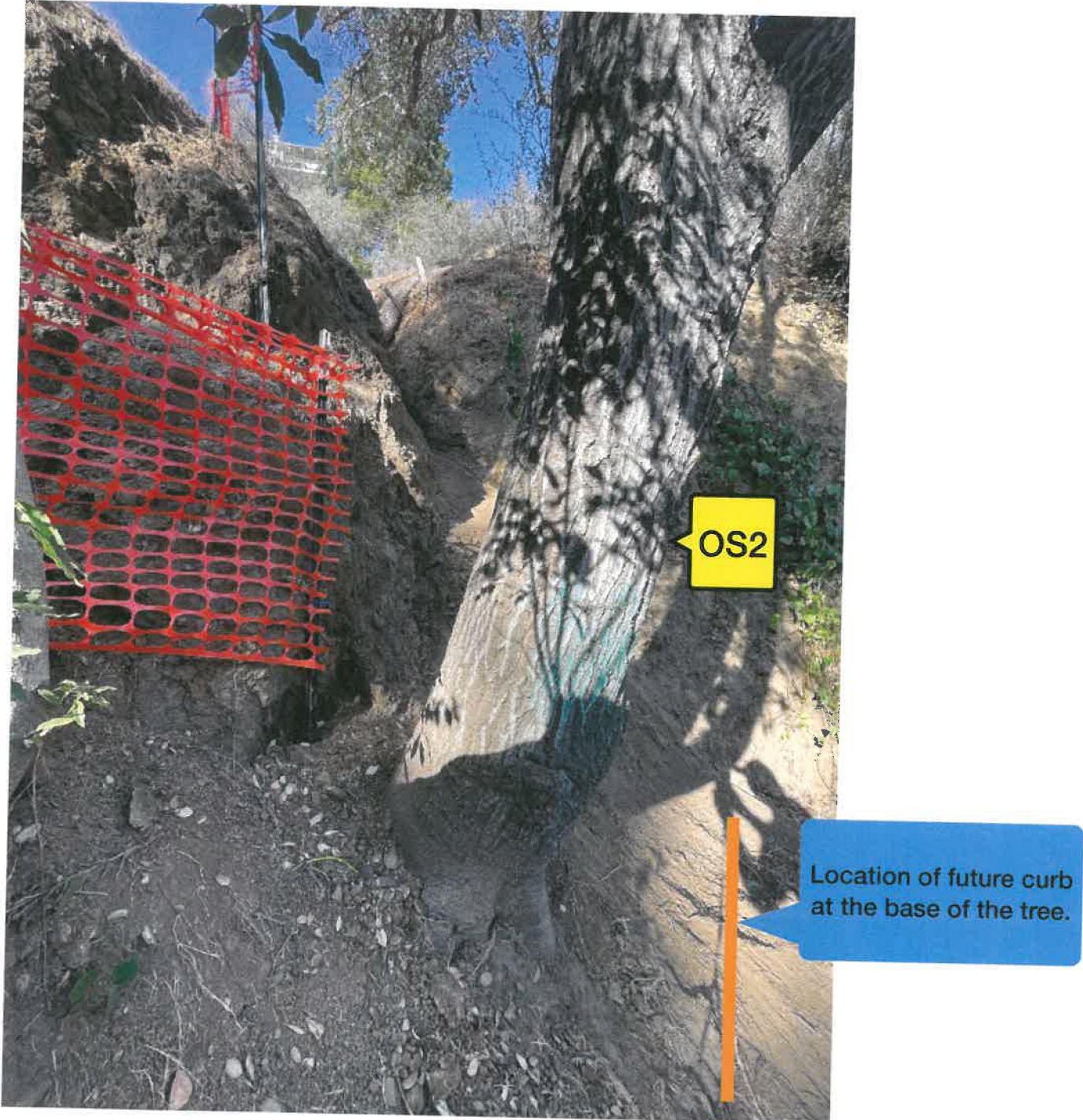
PHOTO 3 - Coast live oak ( Quercus agrifolia ) tree #OS2 is in the public right-of-way will receive minimal impact. Grading will occur approximately 5 feet above the Oak trunk. The road is proposed to be widened with a regular curb to be installed near the base of the tree. If roots are encountered a shallow curb will be installed instead and will be supported by a tube driven into the ground. This tree will be retained and protected in place.
