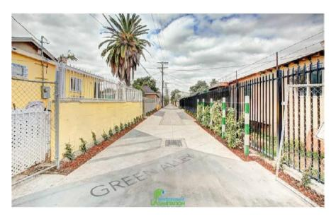
The Avalon Green Alley network in South Los Angeles is a demonstration project for Low-Impact Development (LID) implemented in joint partnership between LA Sanitation and the Trust for Public Land. Two alley segments were identified for full retrofits for stormwater interventions including permeable pavers, dry wells, and rainwater harvesting for plant irrigation.
