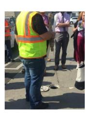
The monitoring wells allow stormwater to collect and be tested for contamination.
