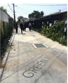
A series of drywells, catch basin intercepts, and permeable surfaces were constructed to capture, infiltrate, and retain stormwater runoff from surrounding tributary areas.
