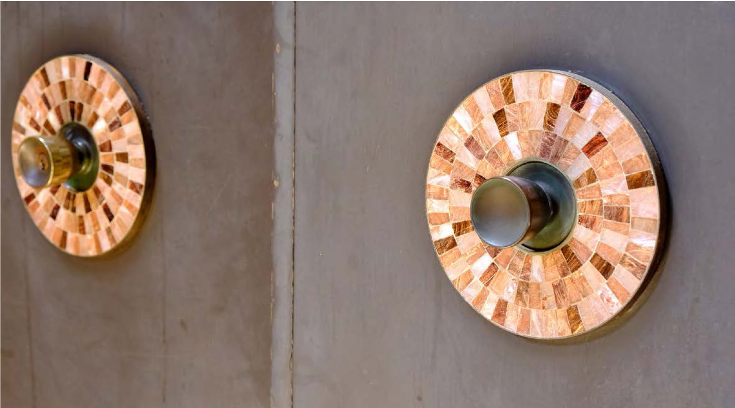
Primary entrance doors. 1335 N. Shadybrook Dr. View west (Luftman 2022)
