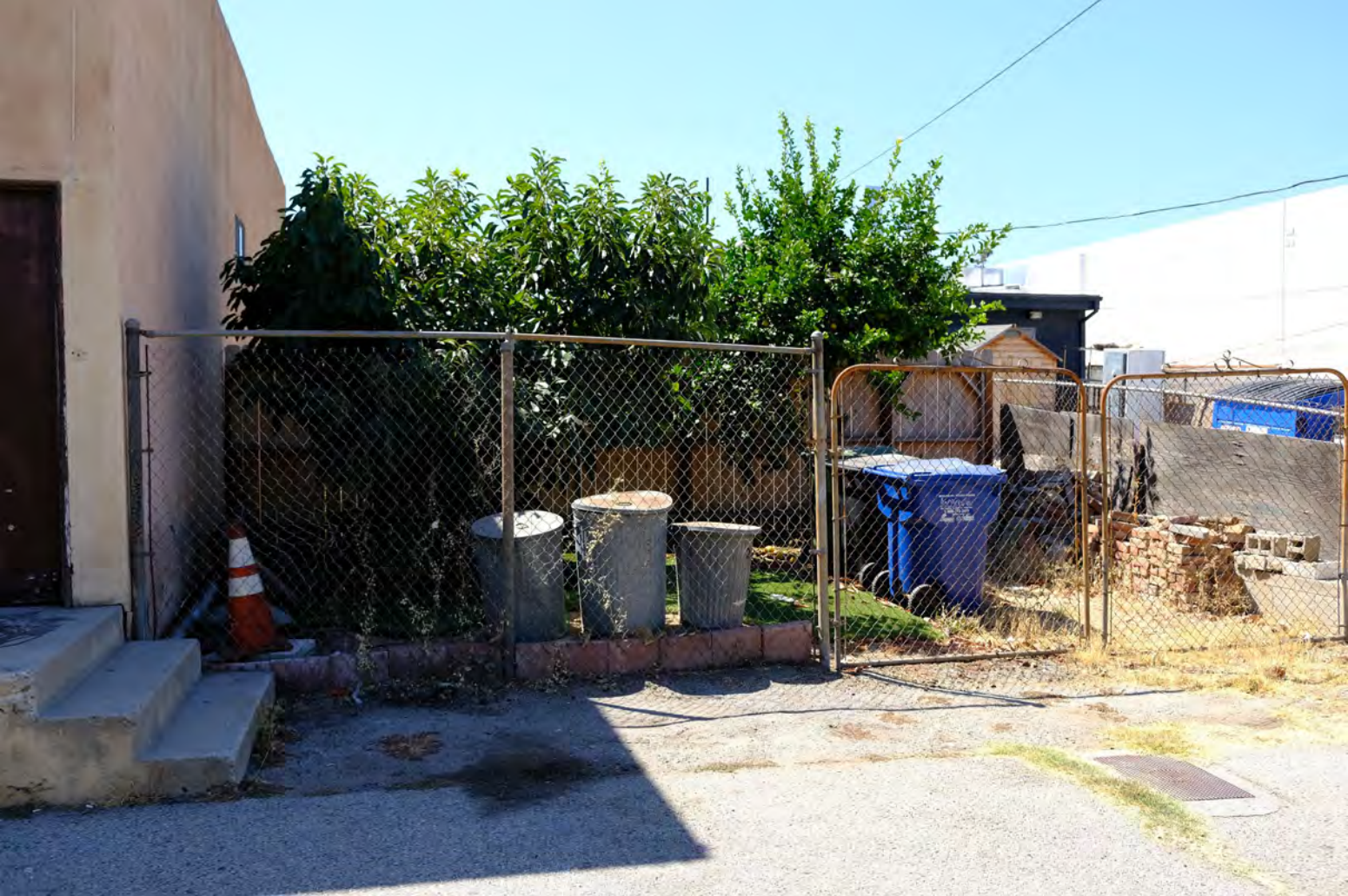
Jay Risk Standard Oil Co. Service Station. View south from the alley. (Luftman 2022)
