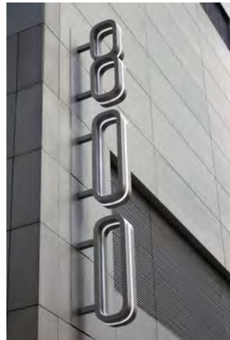
5: 3" DEEP CLEAR ANODIZED ALUMINUM CHANNEL LETTER ADDRESS NUMBER SIGN
