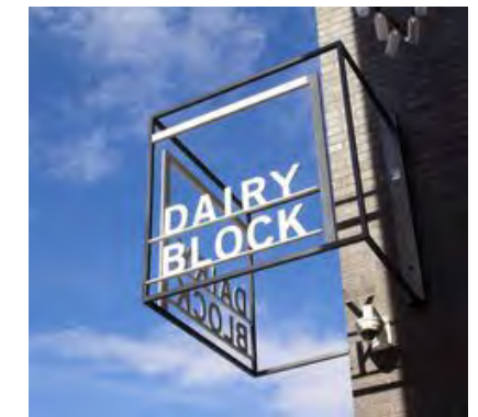
1: CORNER SIGN WITH 1" DEEP STEEL CUT OUT LETTERING, 1'-2" HIGH LETTER
