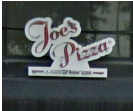
2: CHANNEL SIGN WITH RACEWAY
