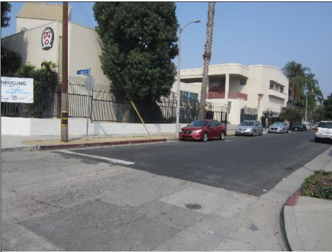
3. Southern side of the subject property.
