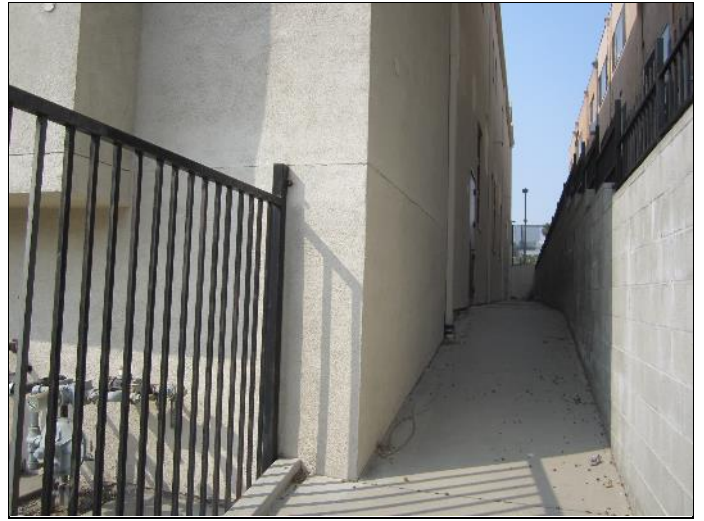
8. Eastern side of the subject building.
