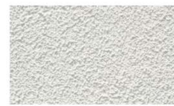
2 CEMENT PLASTER - WARM WHITE - SAND FLOAT FINISH
