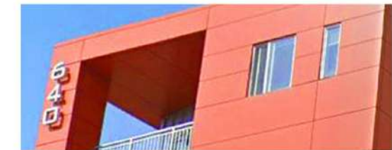
1 METAL PANEL - CUSTOM COLOR "FIRE RED" 9 METAL PANEL TRIM ALL AROUND OPENING - CUSTOM COLOR "FIRE RED" 11 ADDRESS/PROJECT SIGNAGE - WHITE ALUMINUM MOUNTED OUT FROM FACE
