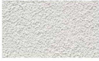
2 CEMENT PLASTER - WARM WHITE - SAND FLOAT FINISH
