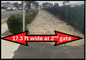
The front setback required to be 20.5 feet is not met— Gate 1 measures 19.3 feet and the fence slopes down to 17.3 feet at Gate 2, placing both segments in clear violation of Performance Standard #4.
