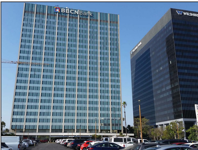
View 5: Looking north across Site's parking structure that will be removed.
