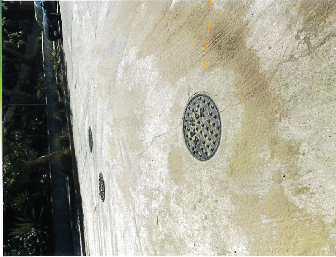
Debris Accumulated around Sewer maintenance. Indication of ponding.
