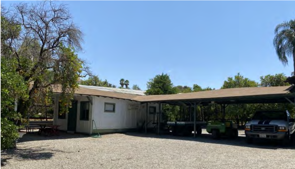
Figure 5: July 2022 view of train station looking southwest from train shed.
