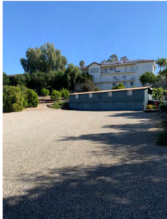
View of Building 9. Grounds are clean and well maintained.
