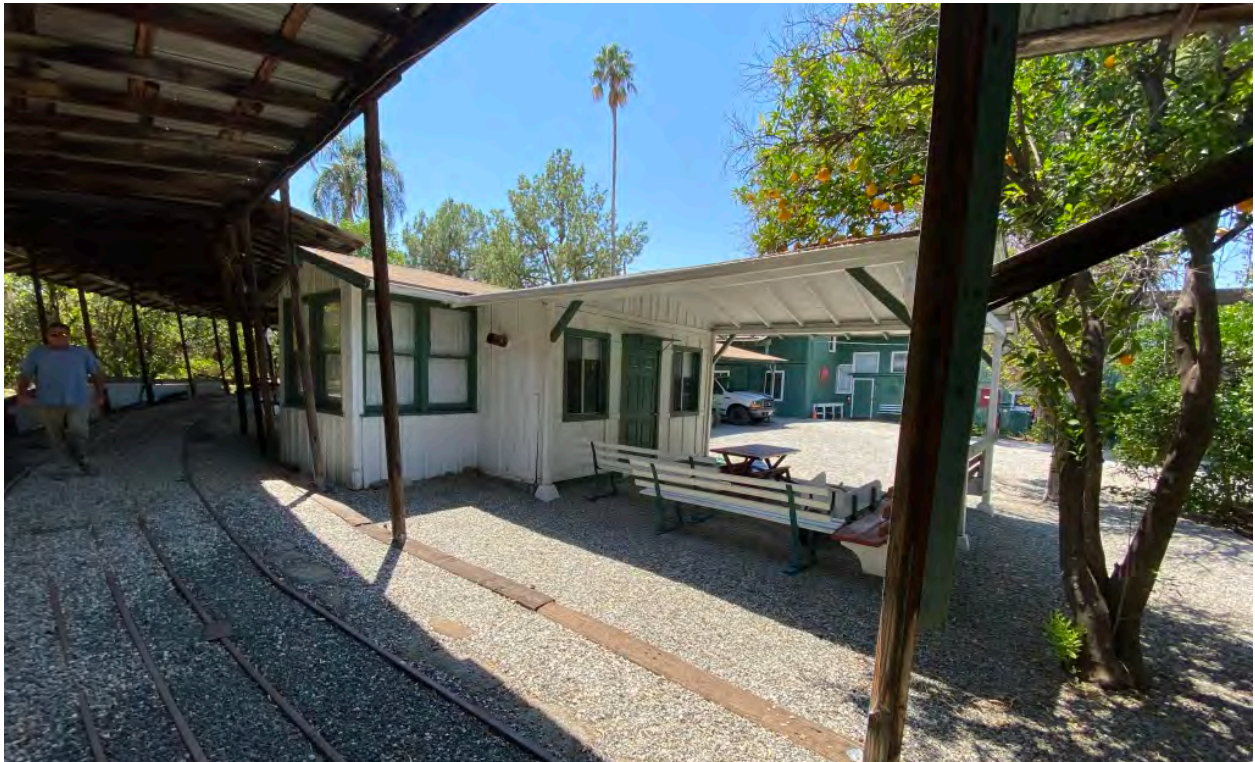
Figure 21: July 2022 view of train station on Project Site looking southwest from train shed.
