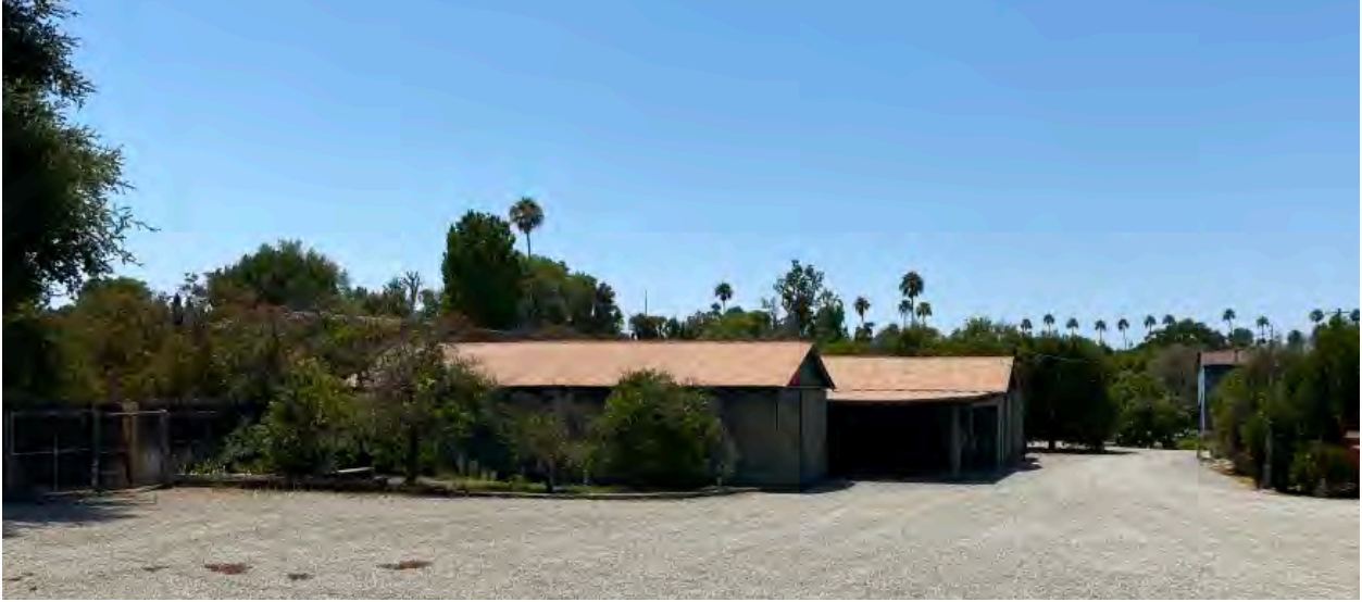
Figure 24: July 2022 view of storage buildings in southeastern portion of Project Site looking west.
