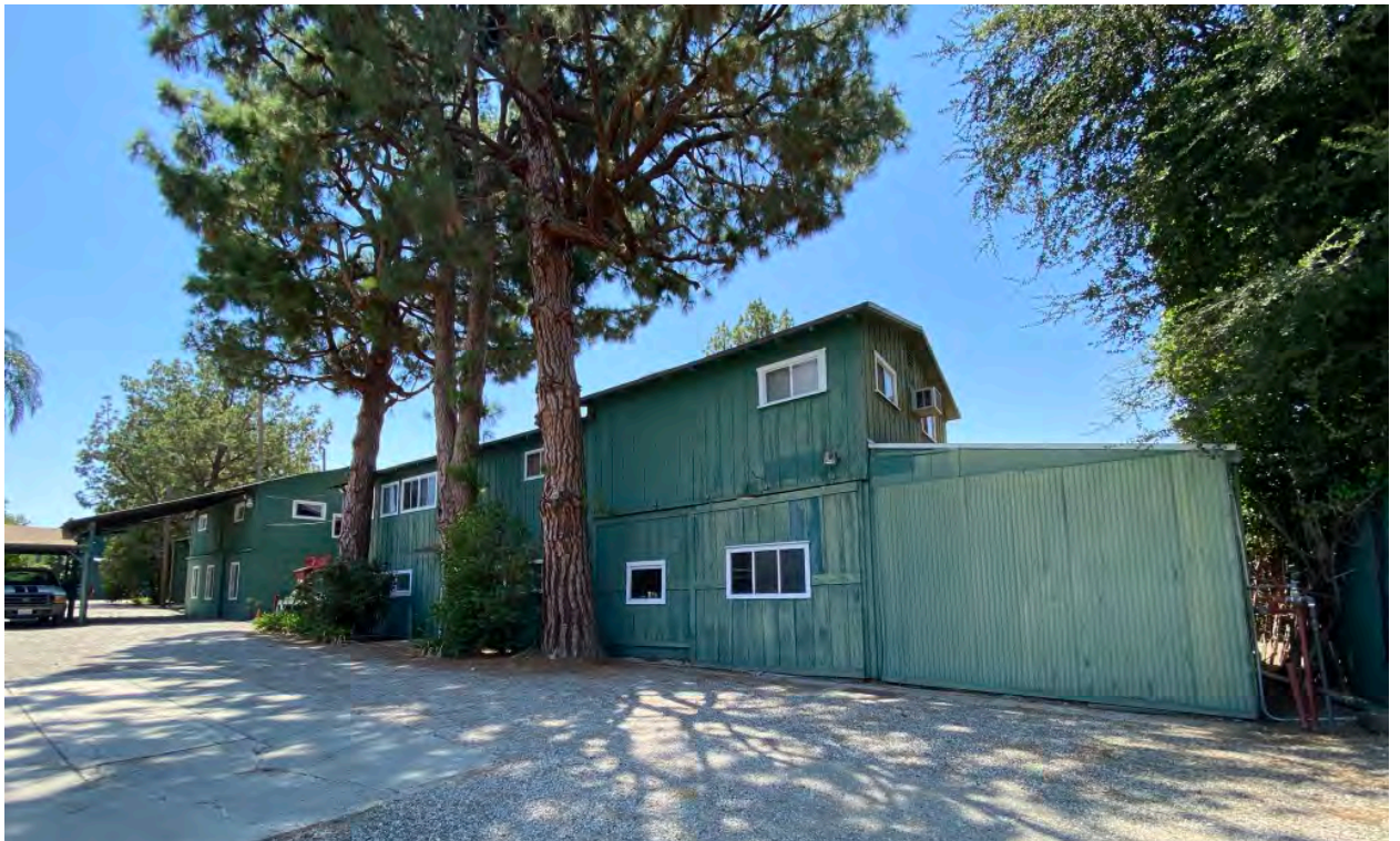
Figure 19: July 2022 view of multi-purpose building on Project Site looking southwest toward east facade.
