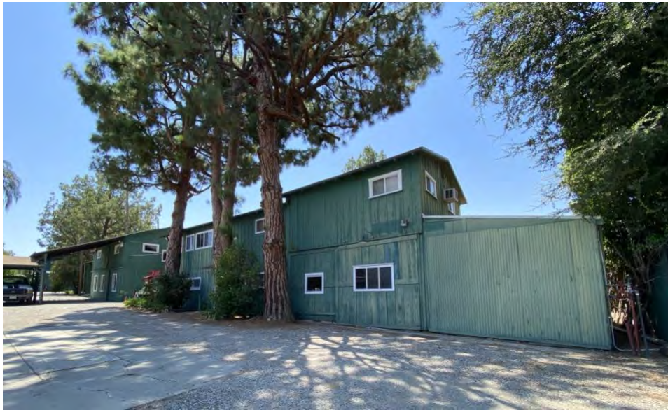
Figure 3: July 2022 view of multi-purpose building looking southeast toward east façade.
