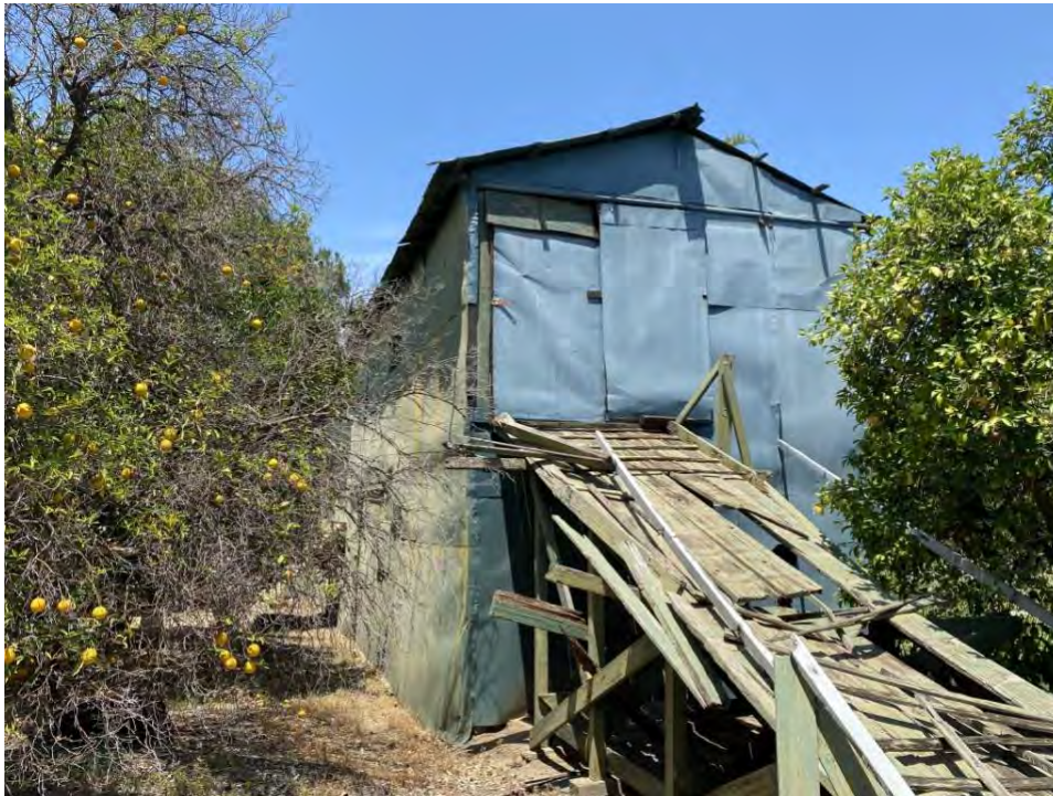
Figure 7: July 2022 view of storage building looking northeast toward south façade.
