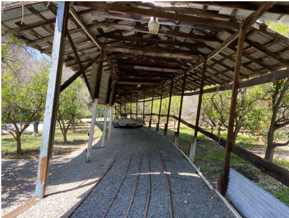
Figure 6: July 2022 view of train shed looking north.
