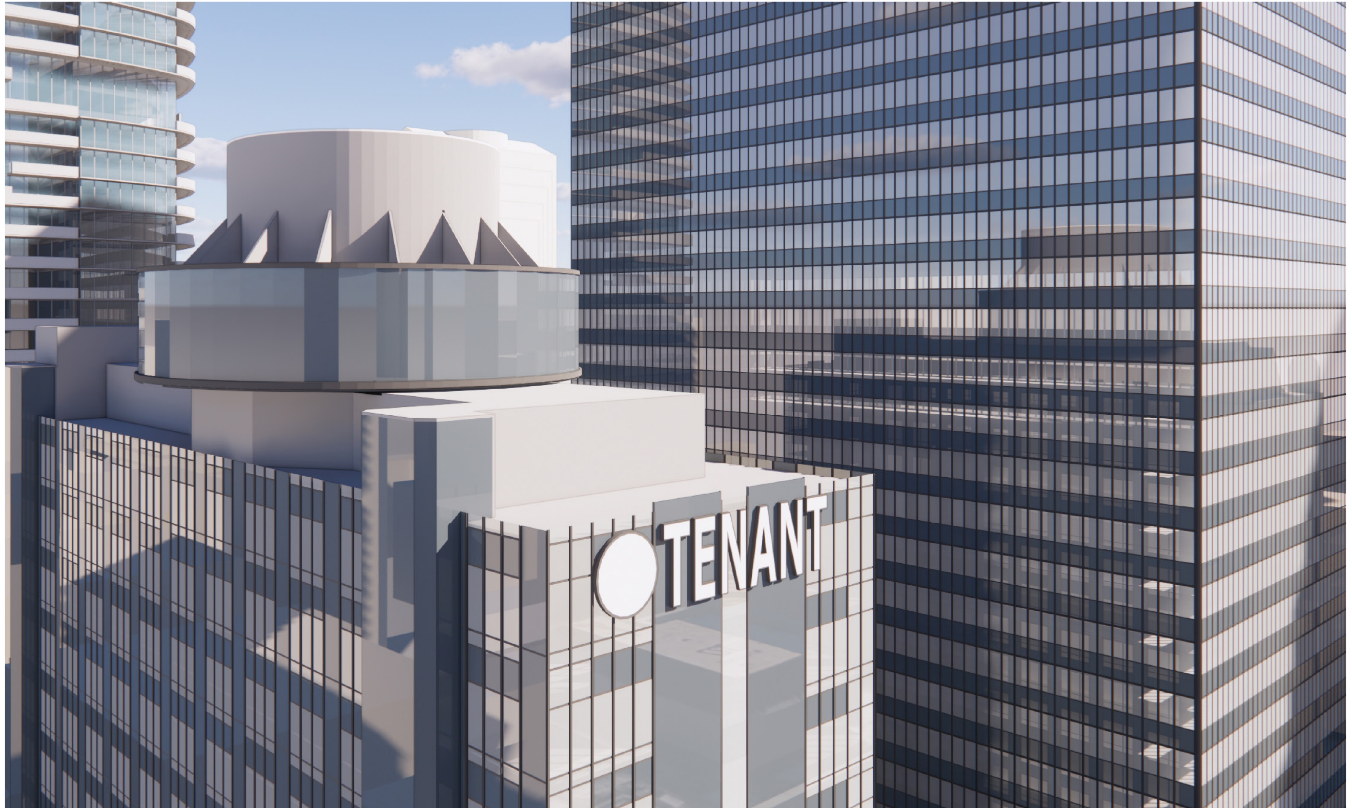
Hotel Tower Top - Facing 7th Street / North
