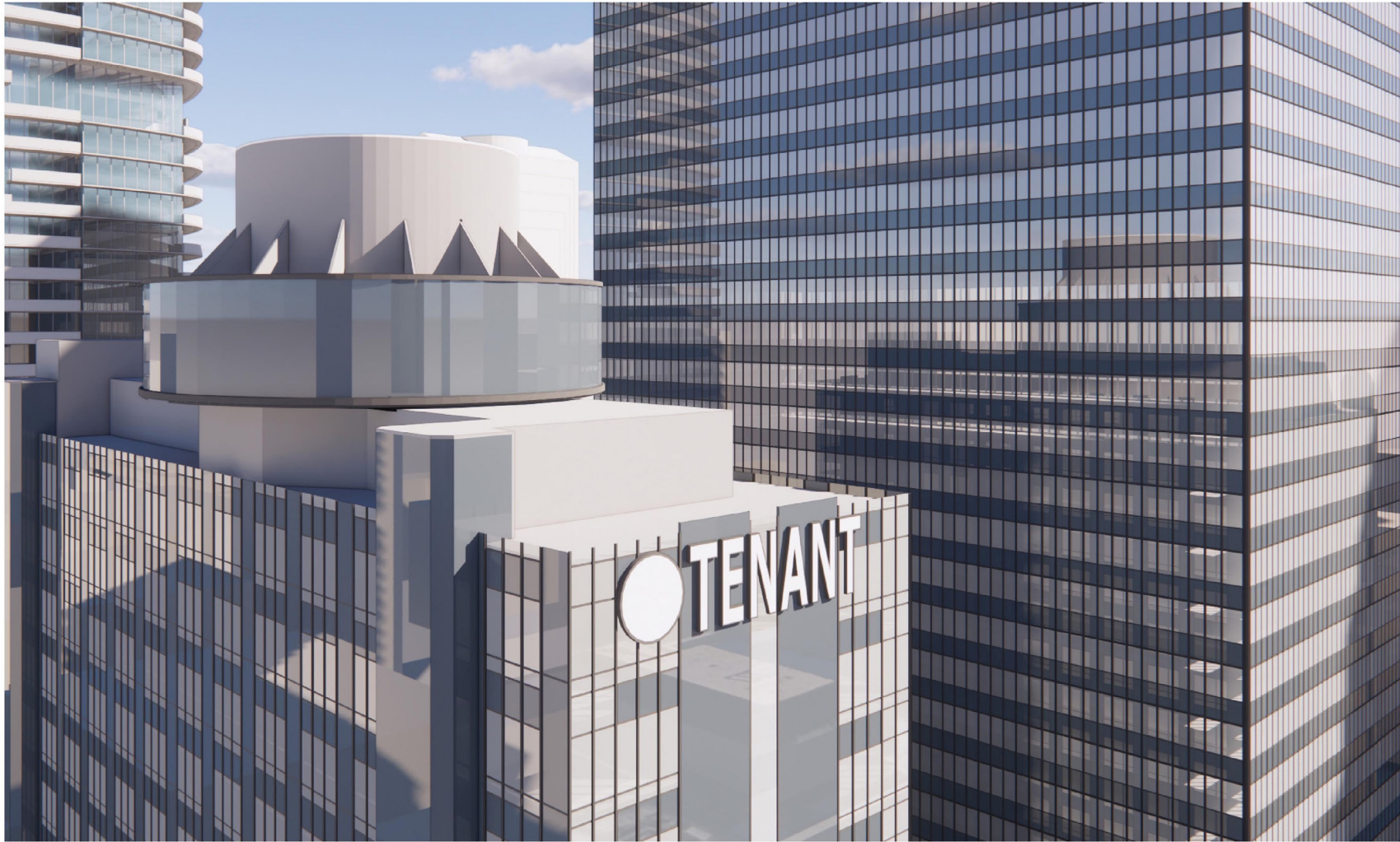
Hotel Tower Top - Facing 7th Street / North
