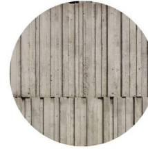
PRECAST CONCRETE WALL
