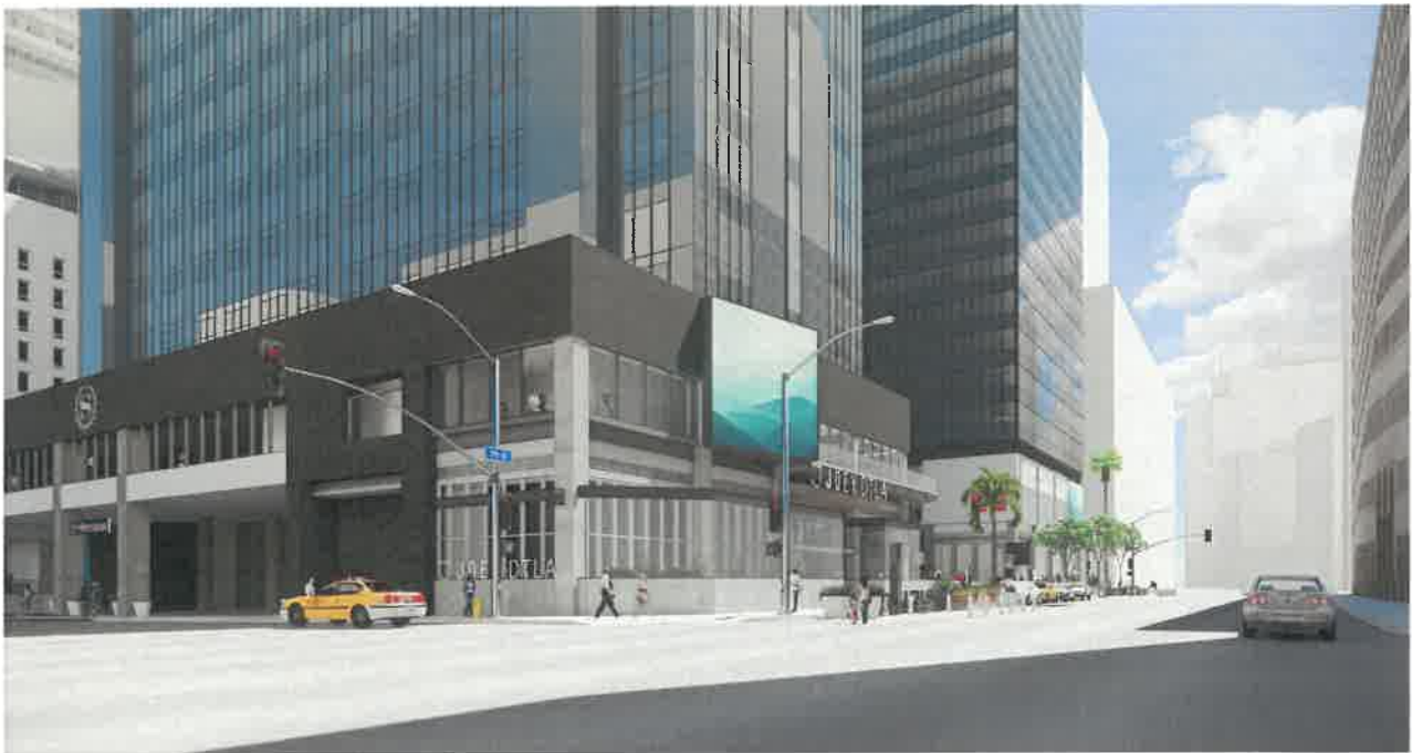
Hope and 7th Corner- Facing 7th Street/ North Facade
