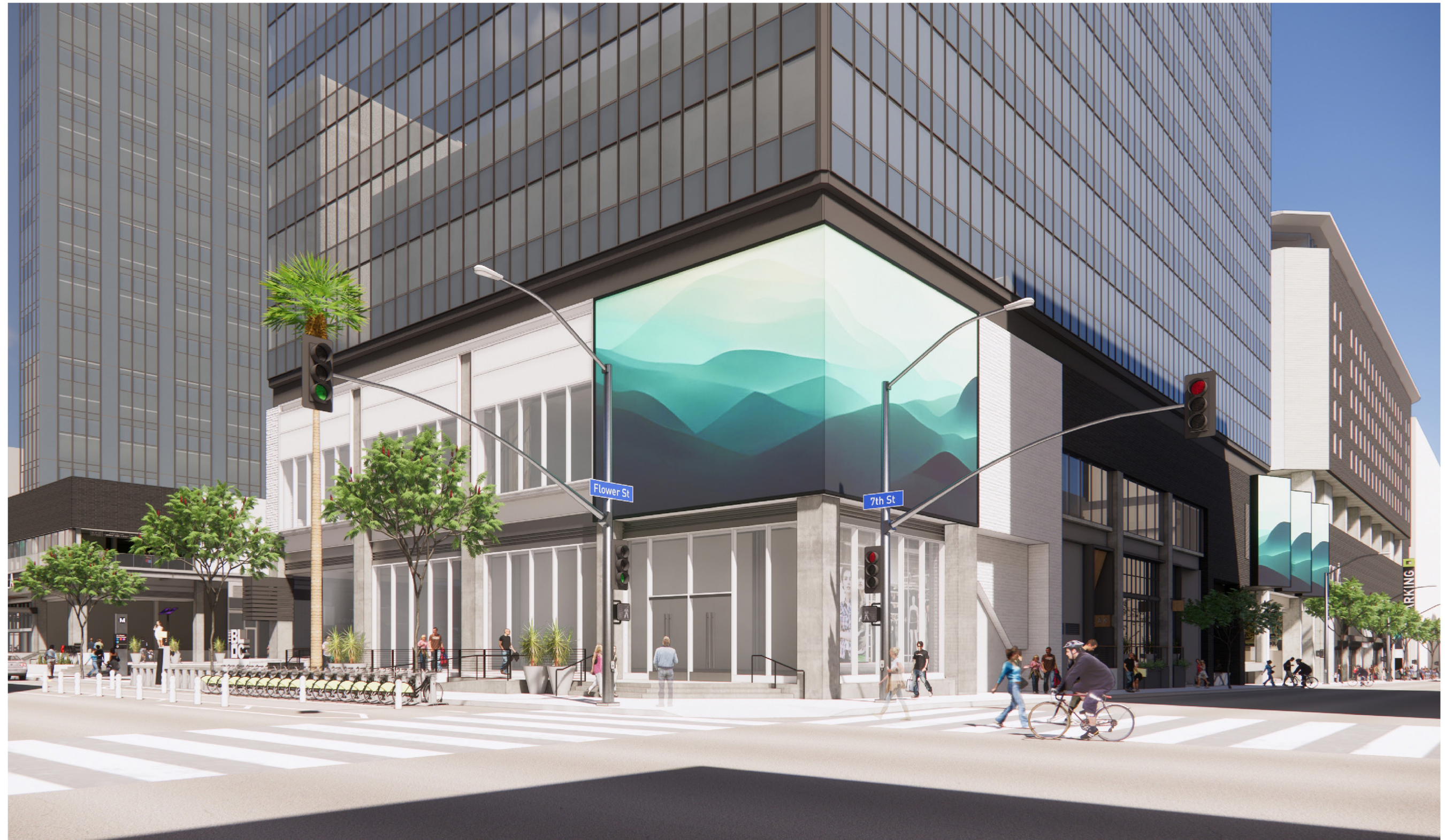
Office Tower Corner - Facing 7th Street/ Northwest Corner
