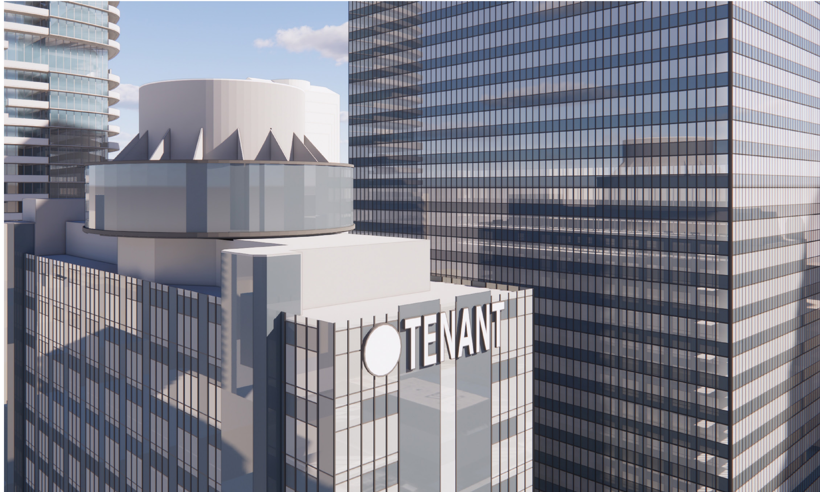
Hotel Tower Top - Facing 7th Street / North
