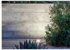
BOARD FORM CONCRETE
