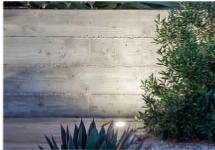
BOARD FORM CONCRETE
