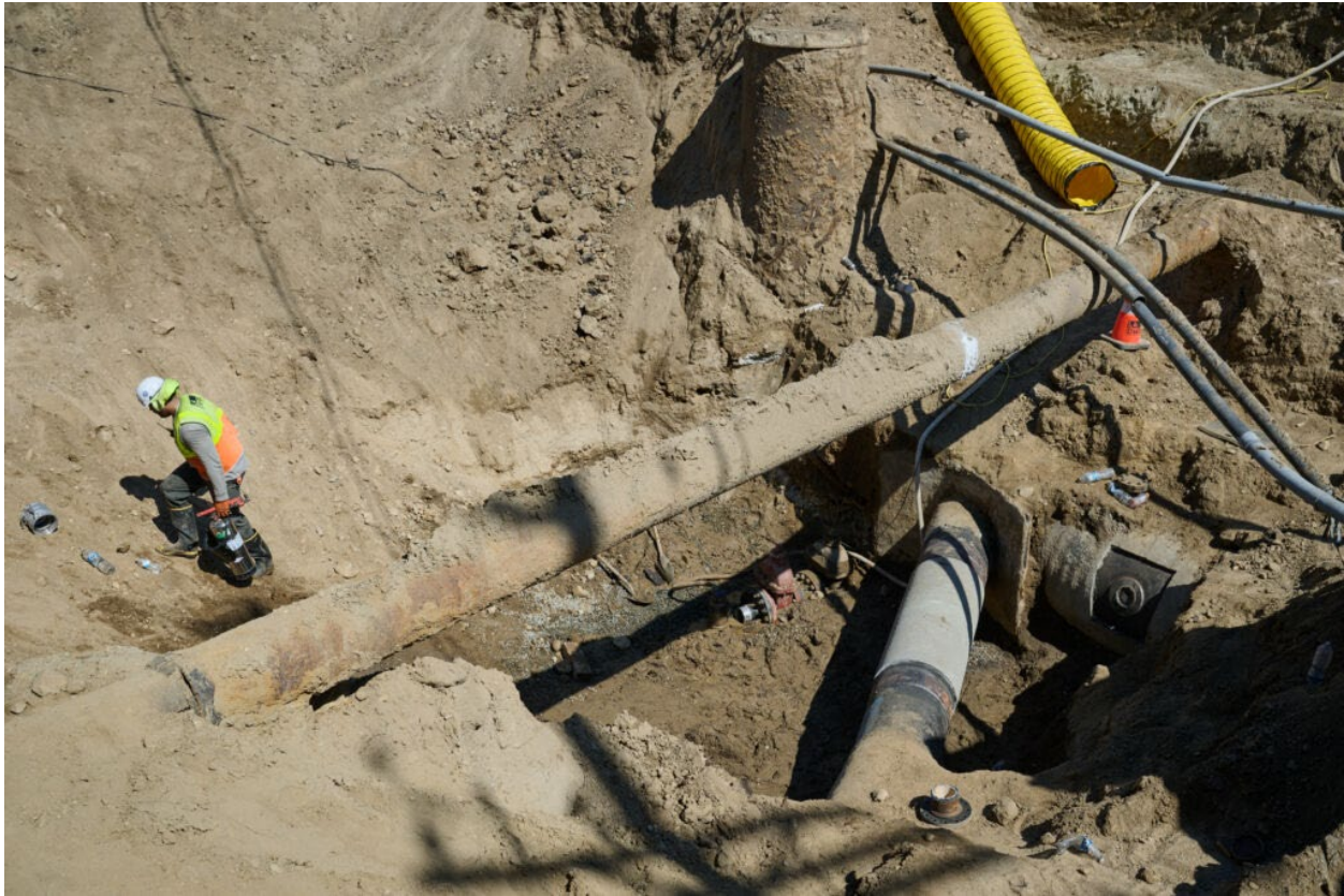
Crews completing excavation (24 feet below ground) and pipe installation
