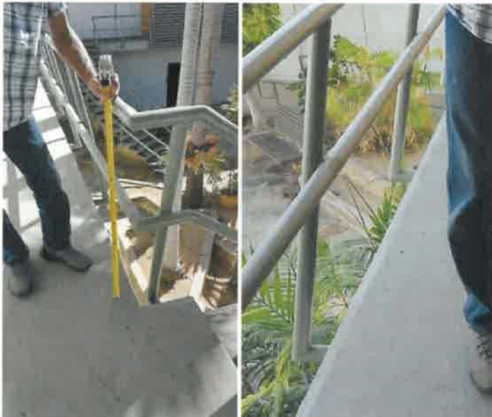
The balcony guard rail height and the lack of the edge protection.
