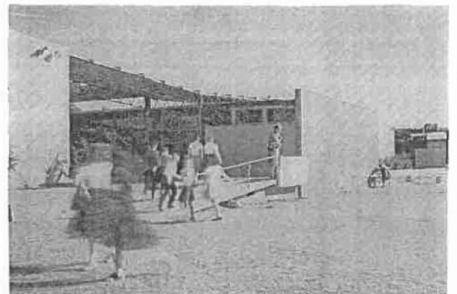
OVERHEAD LOUVERS put shadow on otherwise hot ground plant, easing eye strain, creating livability. Center walkway eliminates passing by classroom window wall, acts as glare control; crossover walkways reduce circulation. Ramps connect two levels of gently sloping site.
