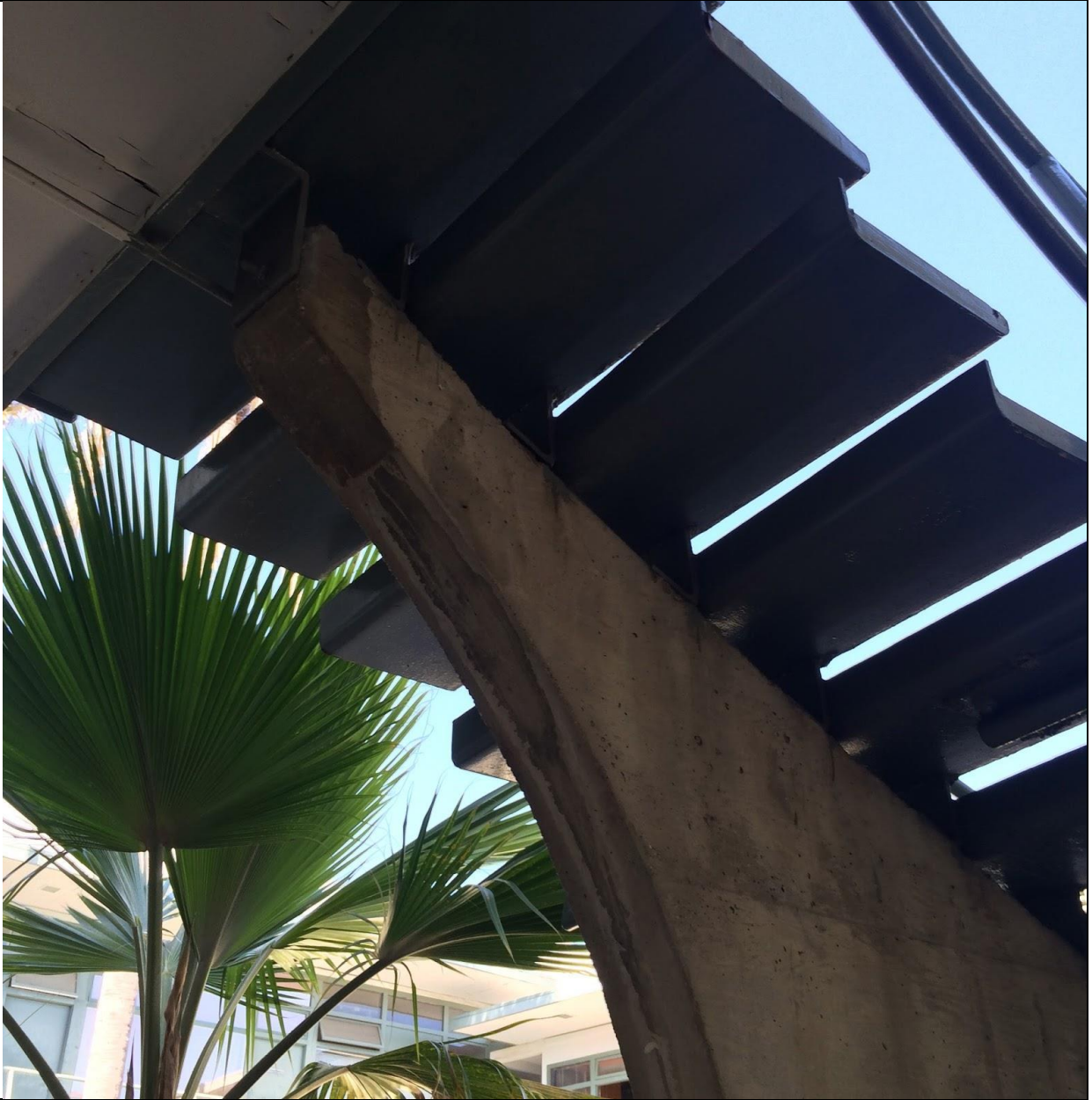
Above: The stairs are cantilevered from a central concrete spine. (photo by Laura Clayton Baker)
