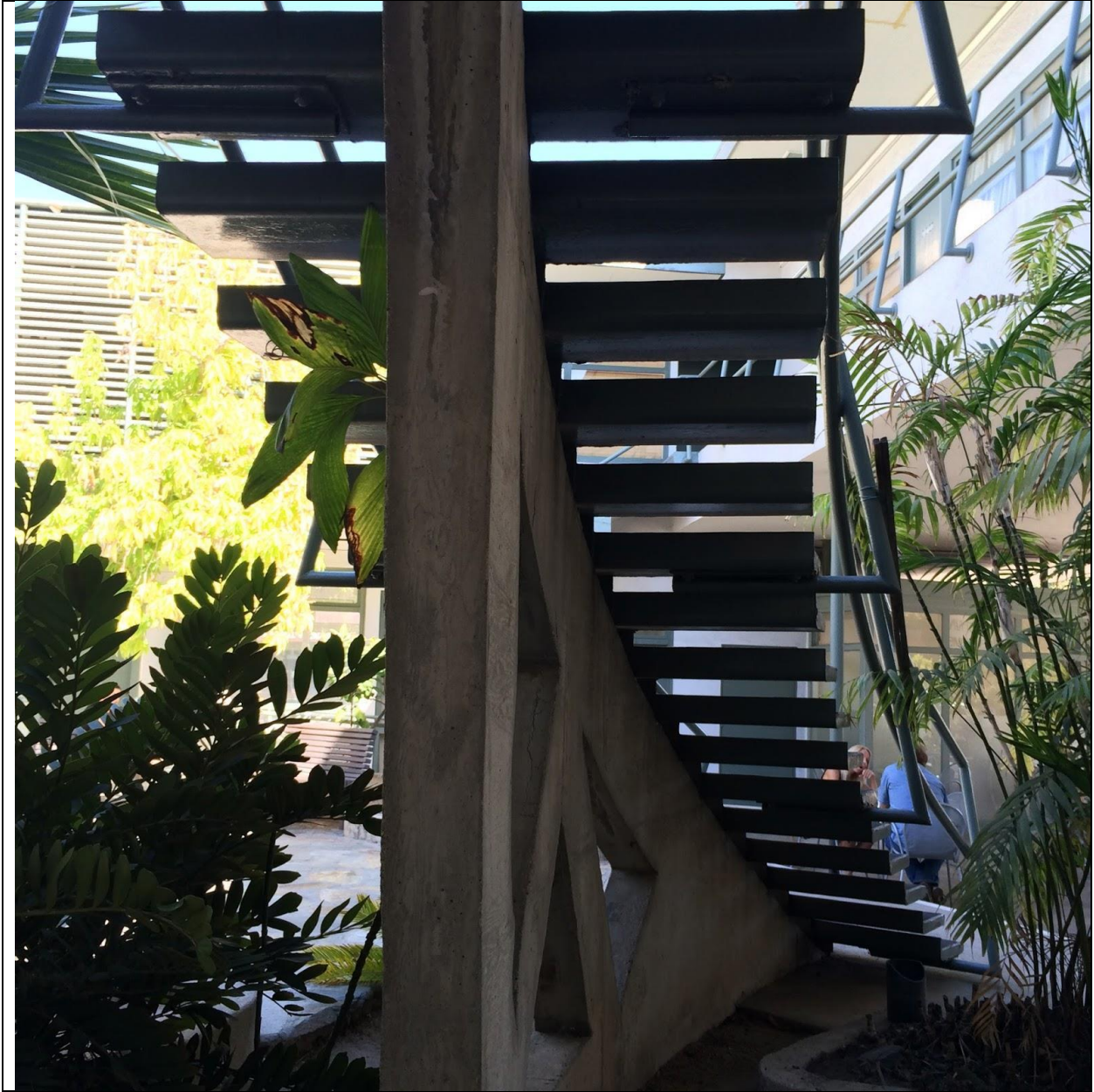
Stairs (Photographic Study) Continued - Above: The stairs are cantilevered from a central concrete spine.
