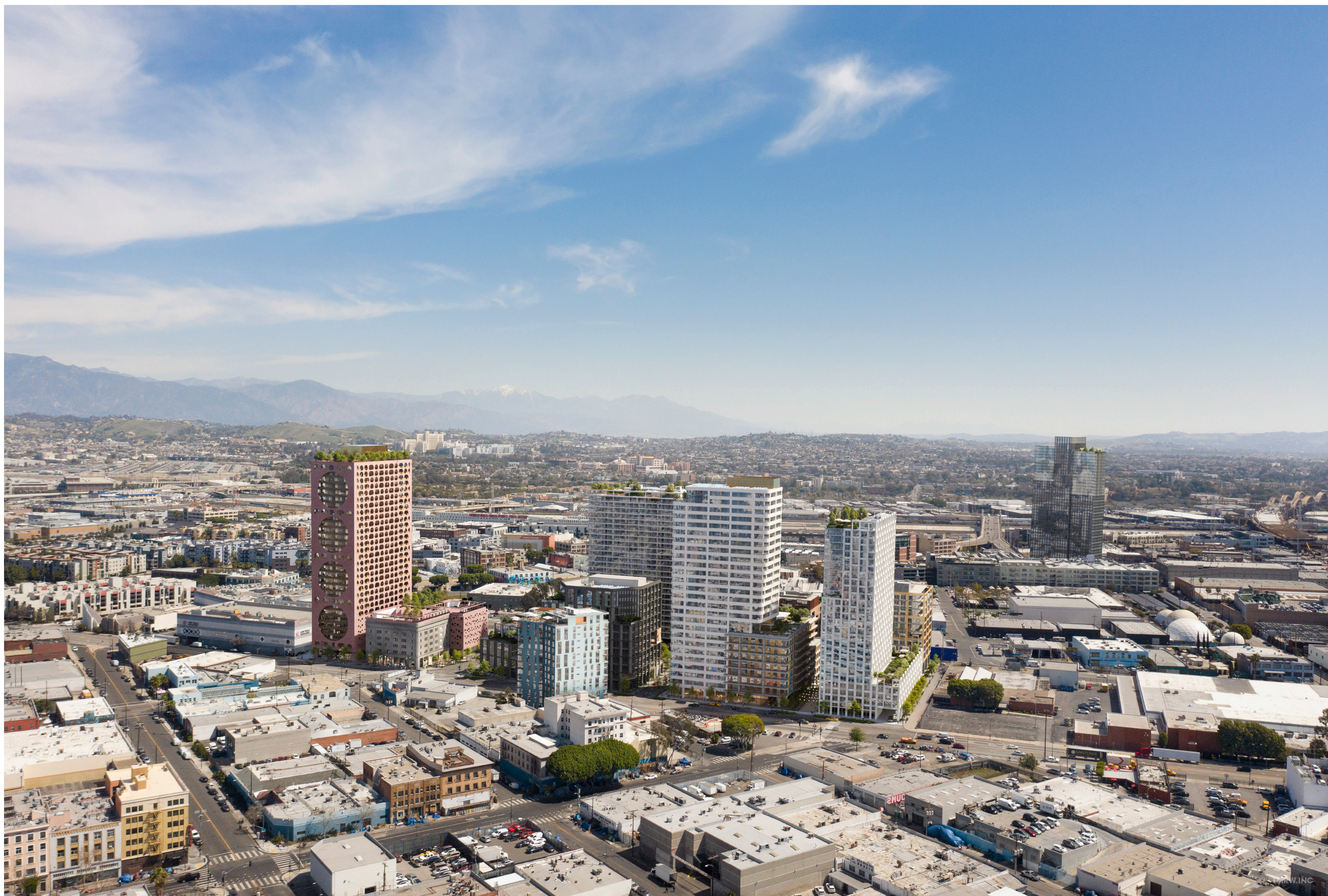
DAYTIME AERIAL VIEW FACING EAST TOWARDS SAN GABRIEL MOUNTAINS
