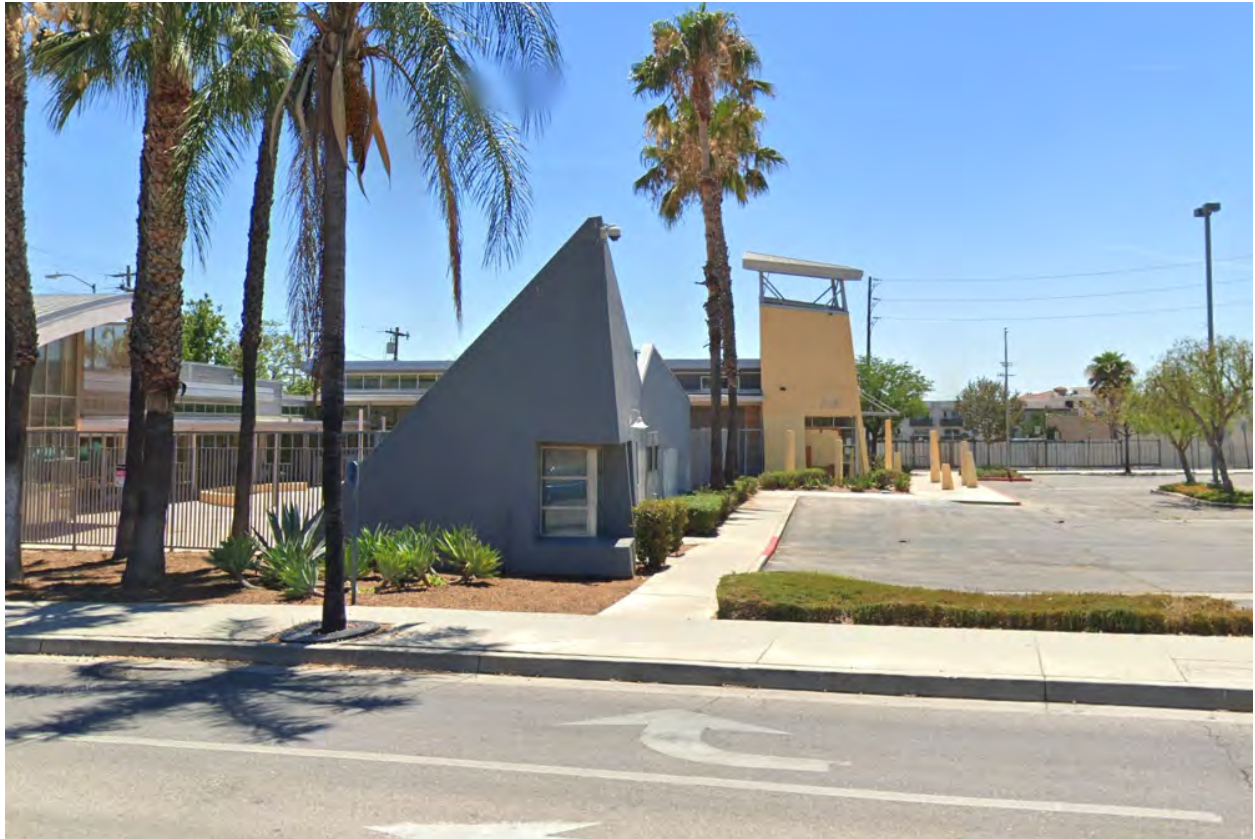
Sylmar/San Fernando Metrolink Station bus operator restroom is located inside the gray triangular building at the center of this photo
