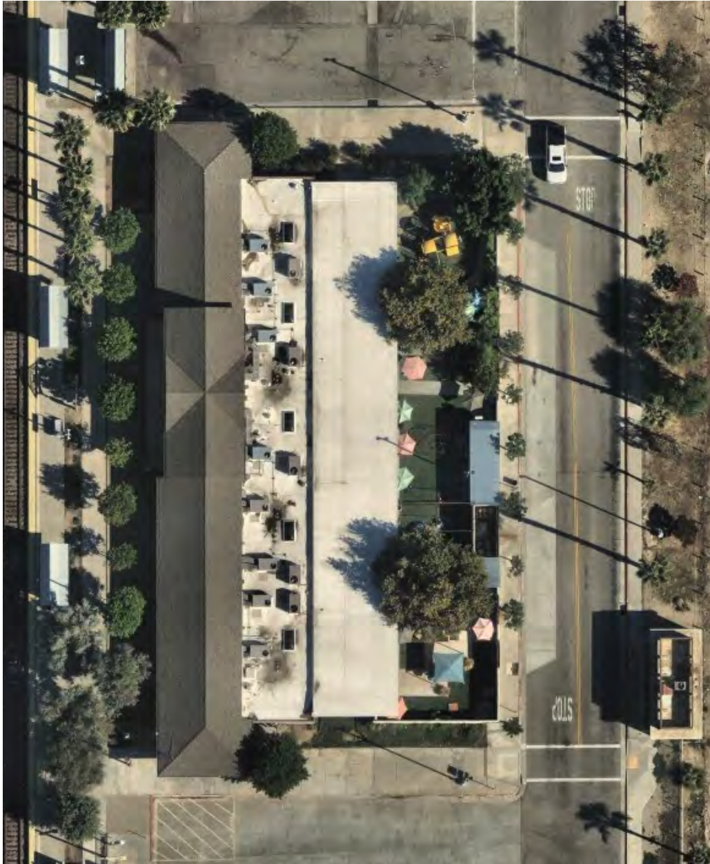
Aerial image of the Chatsworth Metrolink Station Depot
