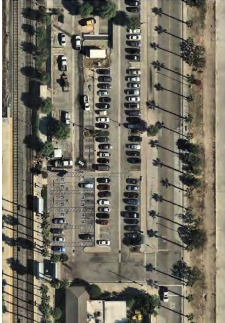
Aerial image of southernmost portion of Parking Lot B; Depot building is to the south
