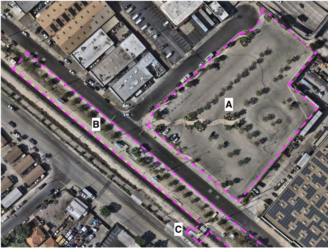
Aerial Image of Sun Valley Metrolink Station (Areas covered by this RFP are outlined in pink and labeled) A. Parking Lot; B. Platform; C. Pedestrian at-grade crossing. Landscaping is throughout.
