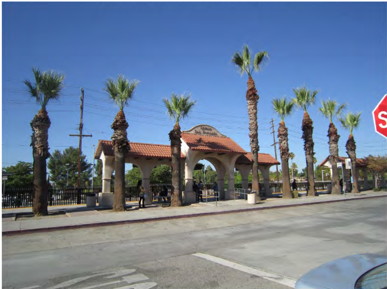
Figure 2.9 Sylmar/San Fernando Metrolink Station
