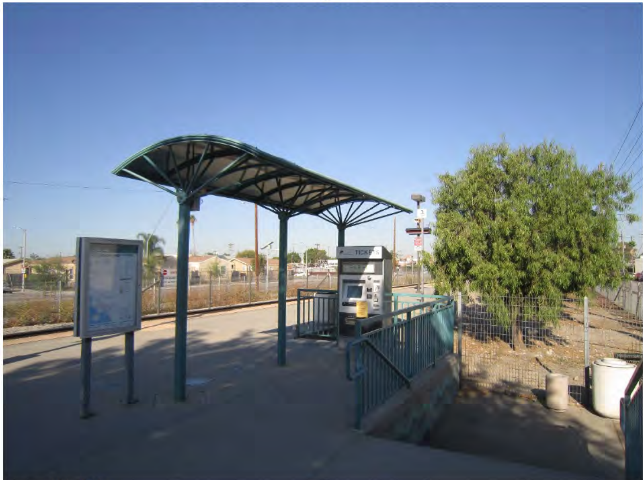
Figure 2.8 Sun Valley Metrolink Station
