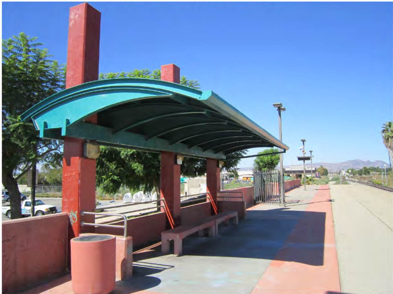
Figure 2.7 Northridge Metrolink Station
