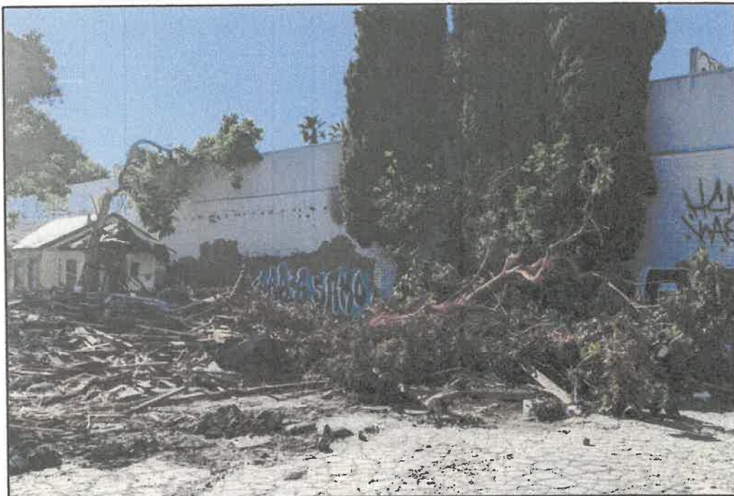
Photograph 8. Building 6 overview (demolished), view southwest
