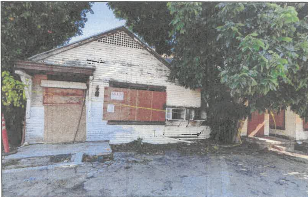
Photograph 4. Building 3, western façade, view southeast
