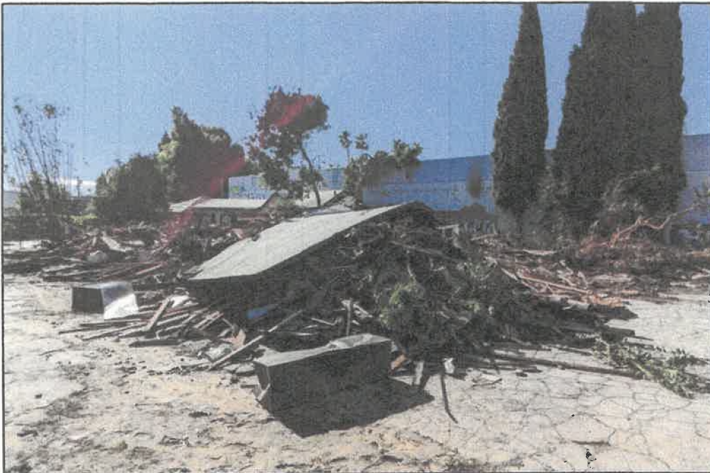
Photograph 7. Building 5 overview (demolished), view southwest
