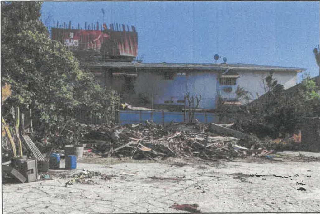
Photograph 1. Building 1 overview (demolished), view east.
