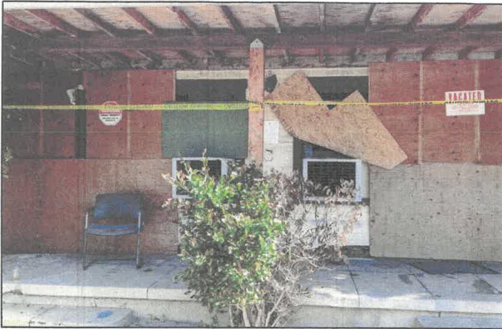
Photograph 3. Building 2, closeup of western façade, view east
