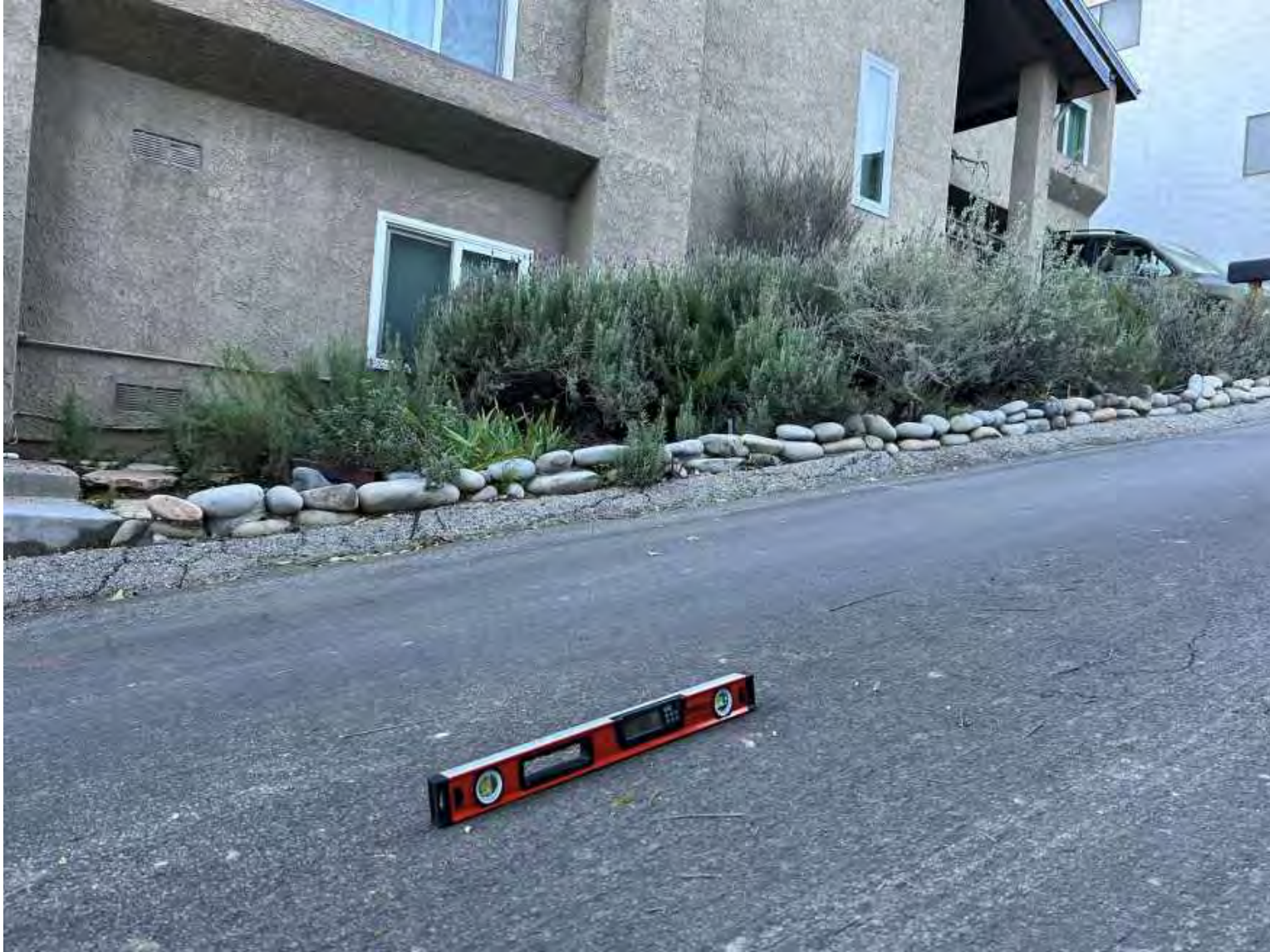
Exhibit 3.8: Photograph of Digital Level In Front of 21318 Las Pitas Road
