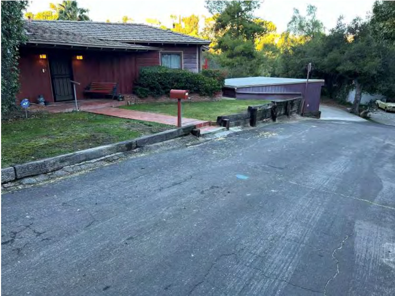
Exhibit 3.6: Photograph of Las Pilas Road Looking Westward
