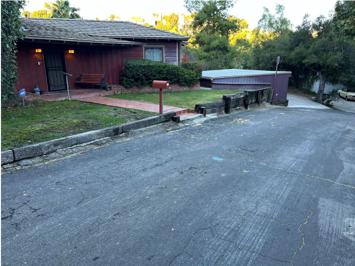
Exhibit 3.6: Photograph of Las Pilas Road Looking Westward
