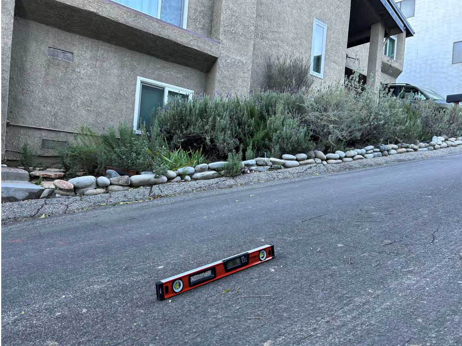
Exhibit 3.8: Photograph of Digital Level In Front of 21318 Las Pilas Road
