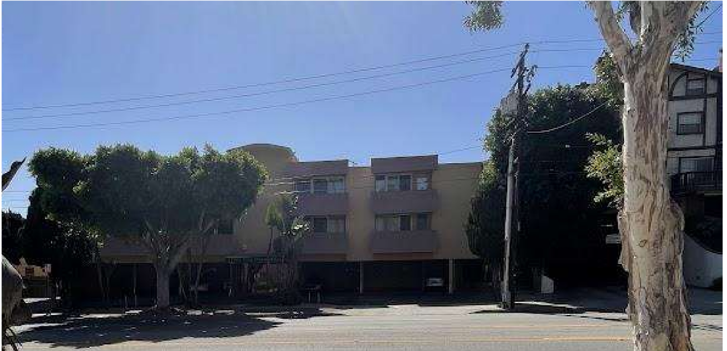
3-Story multi family building across Stocker St., in the County of Los Angeles, facing South.
