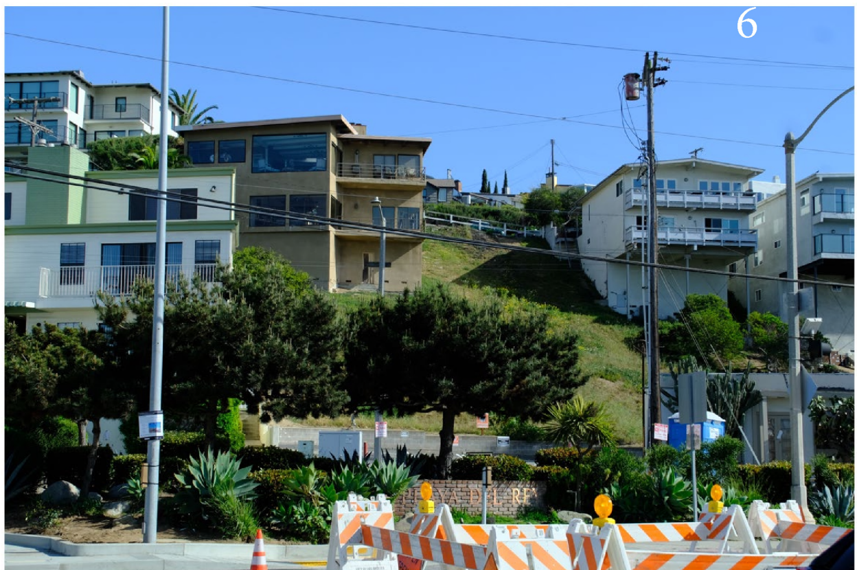
Looking south towards the lot from Culver Boulevard
