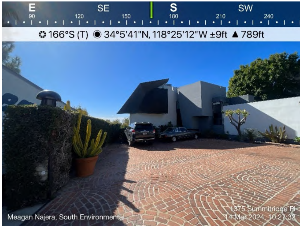
Image 3.) View of the Project Site towards the south from the gate entrance into the property.
