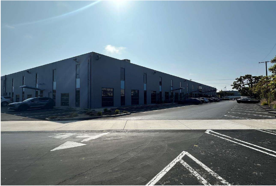
13. View of project site facing West.
