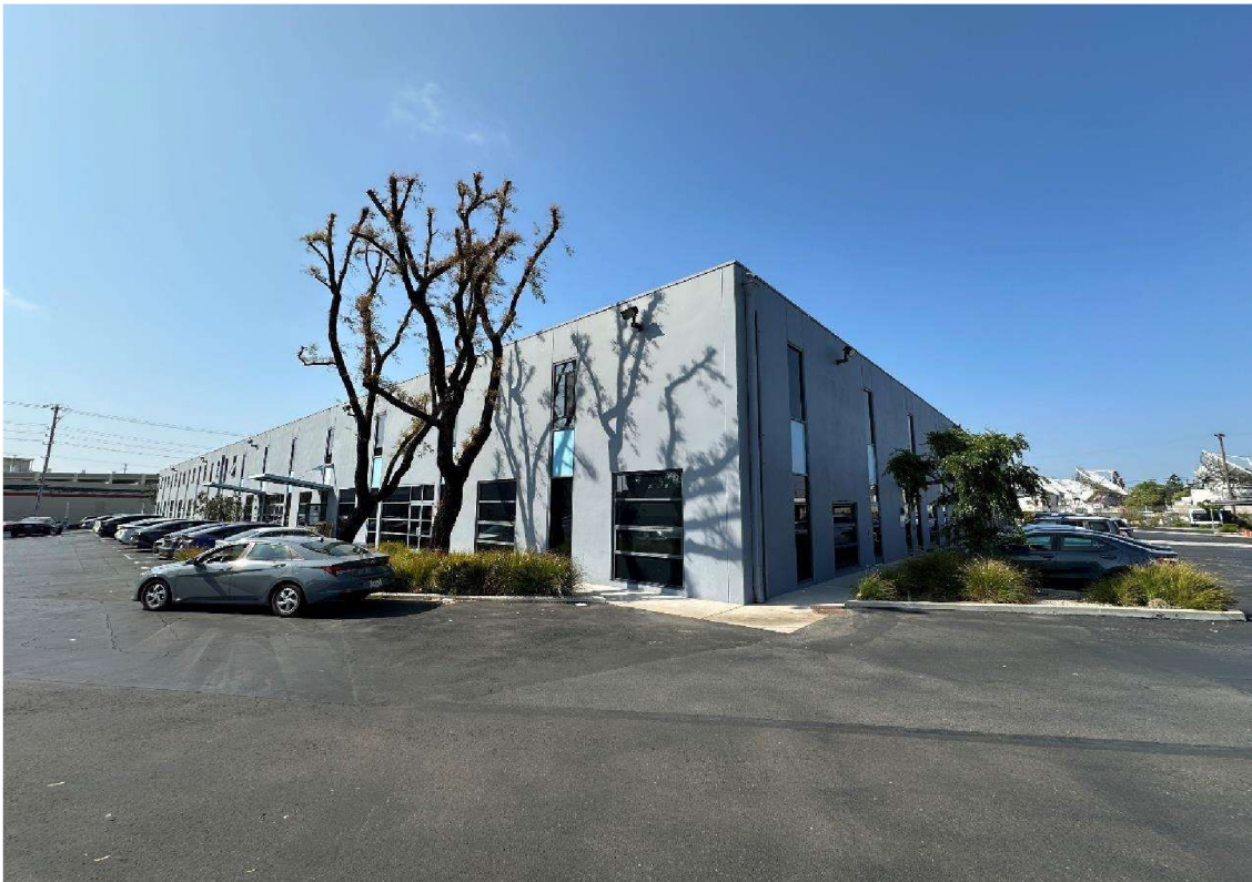
4. View of Project Site facing Northwest.
