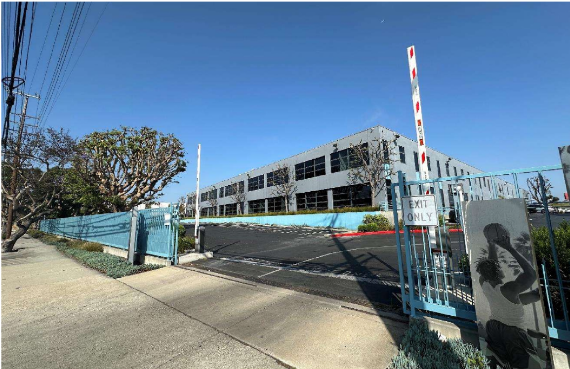
6. View of Project Site facing Northeast on Culver Blvd.
